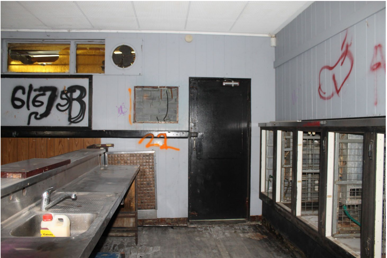
View 55 Door leading to the service yard from behind the counter
