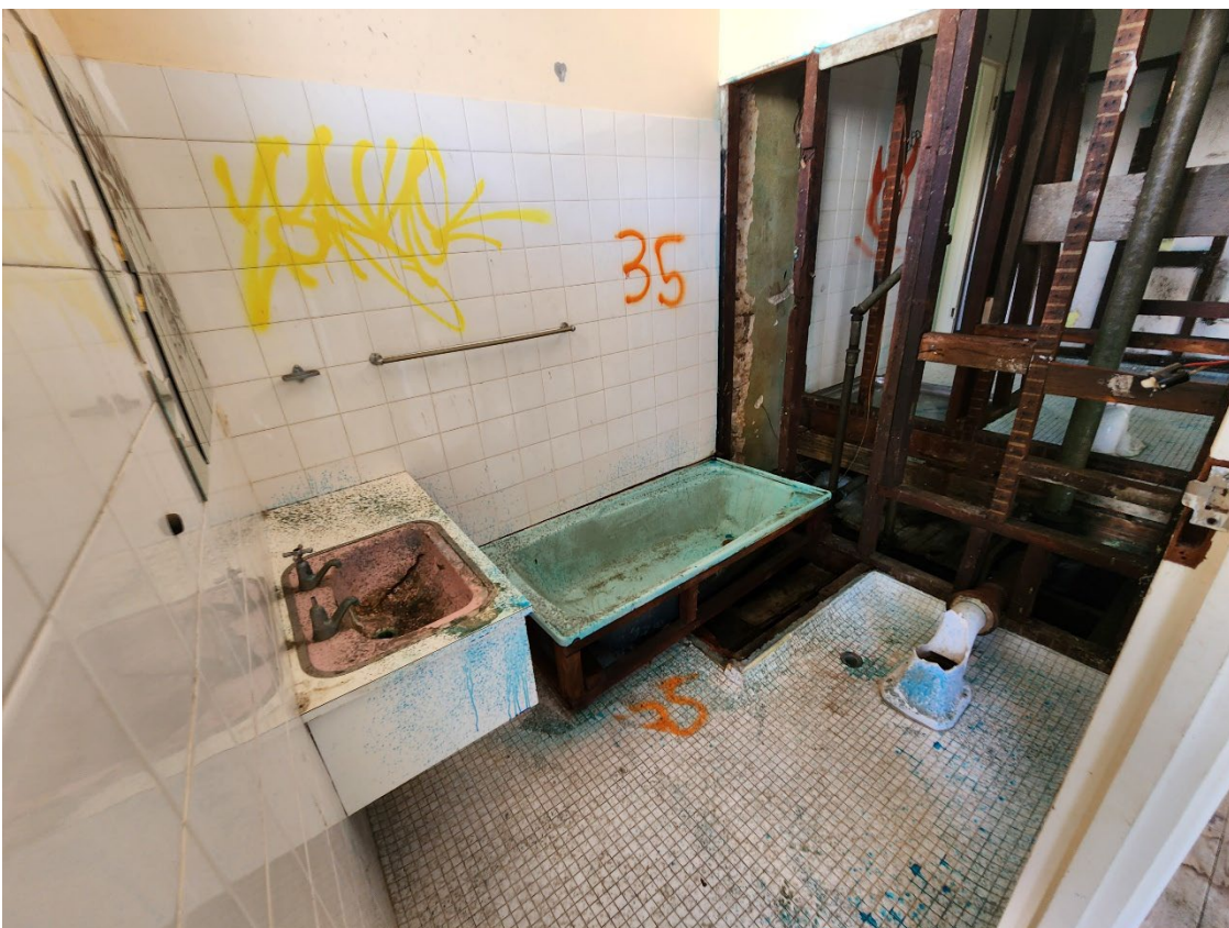
View 82 Interior of Room 3 bathroom
