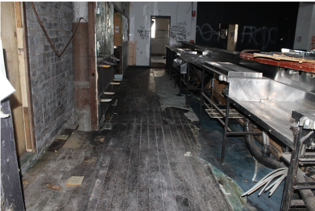
View 40 Timber floorboards and steel benchtops behind the counter
