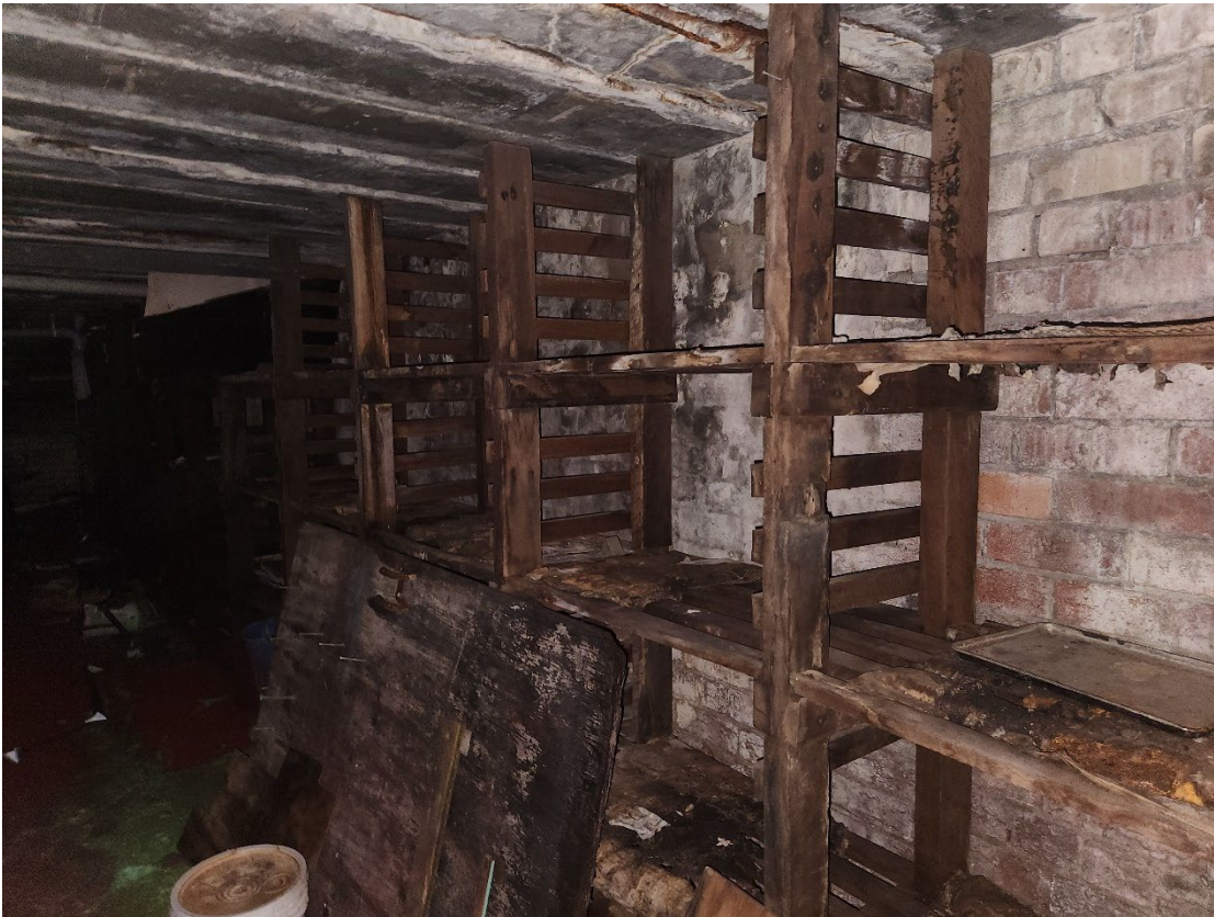
View 112 Remnant timber shelving in the basement
