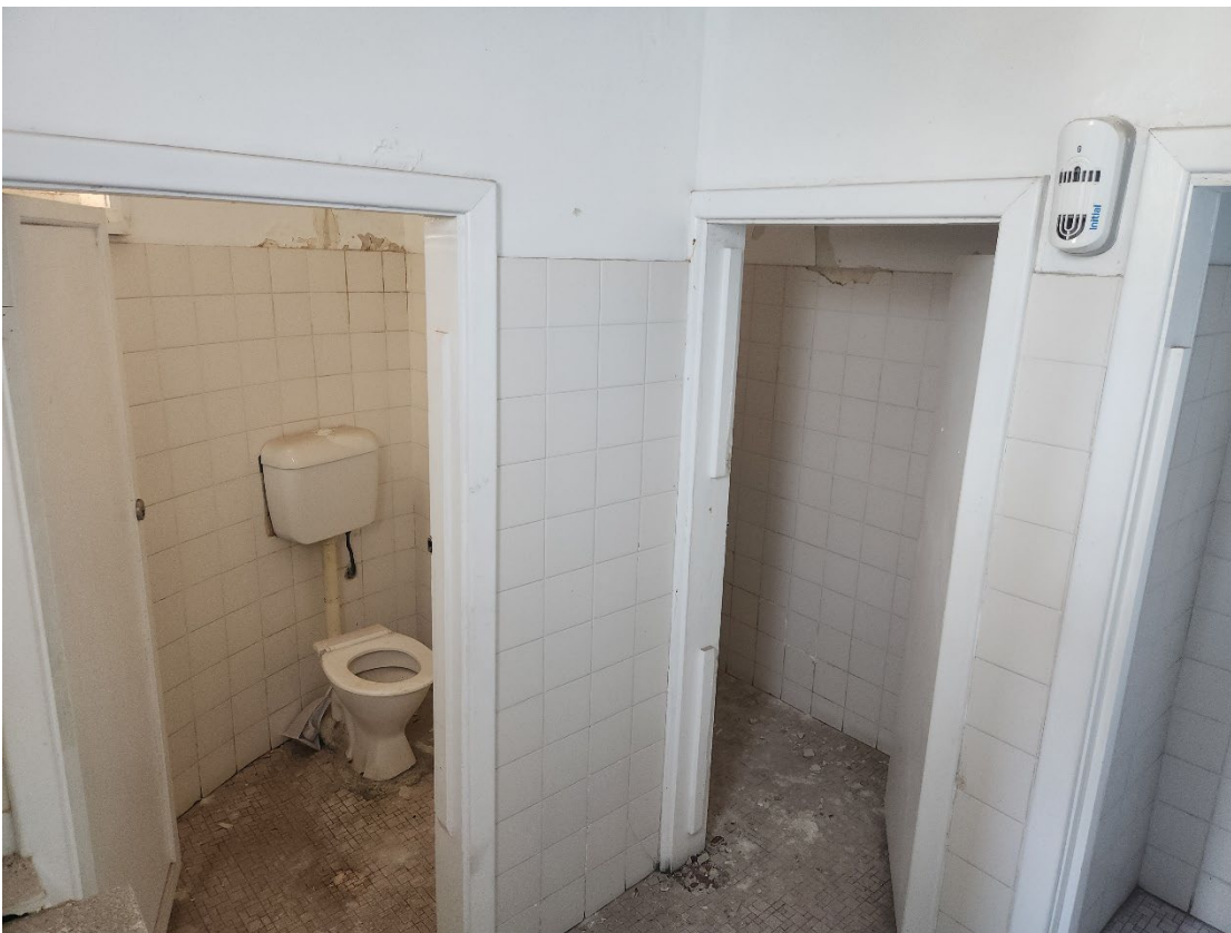
View 50 Tiling to toilet floor and walls
