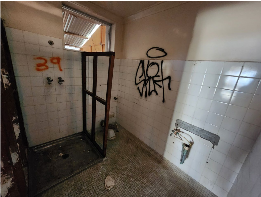
View 91 Existing toilet in the Laundry
