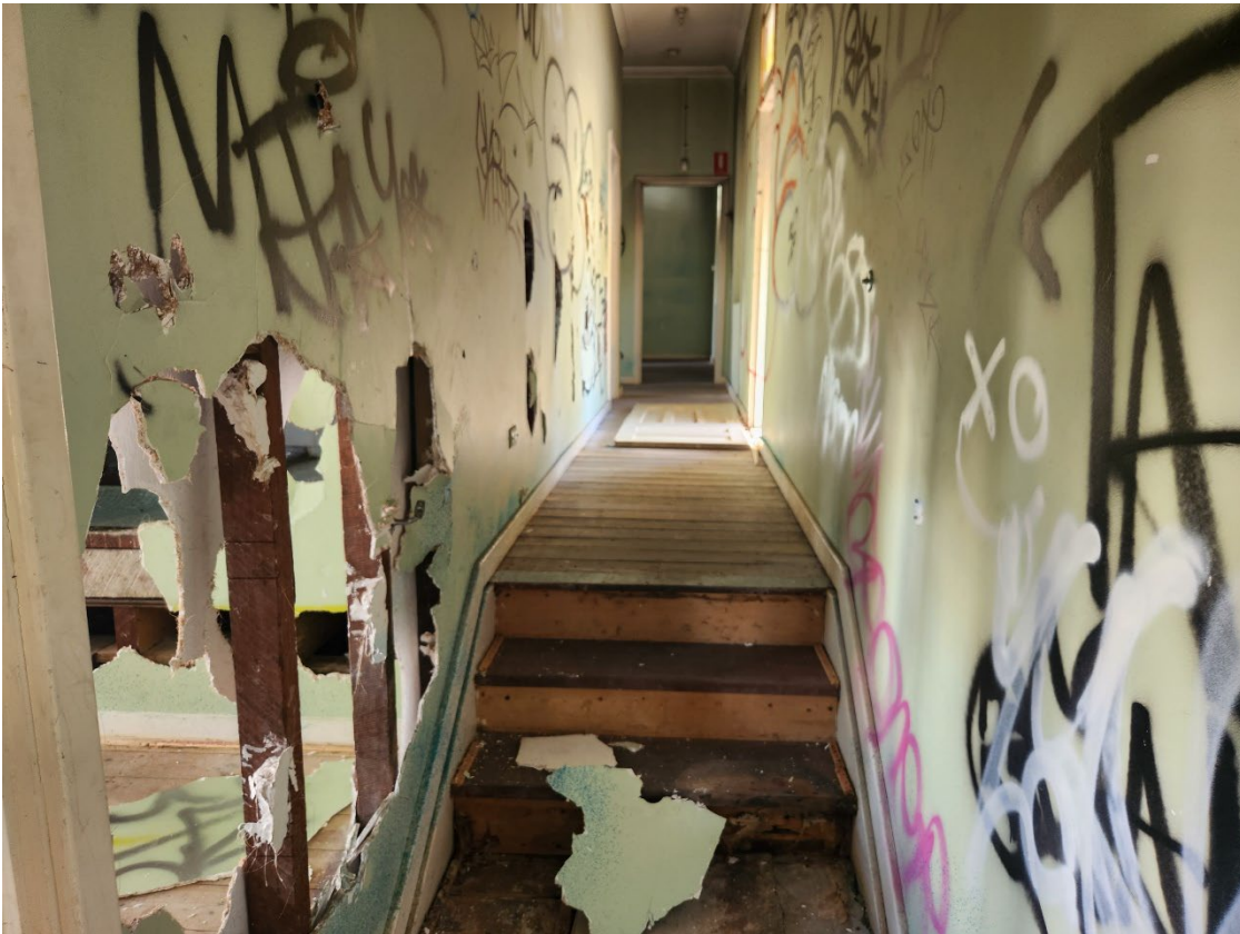
View 83 Hallway steps where the floor level changes
