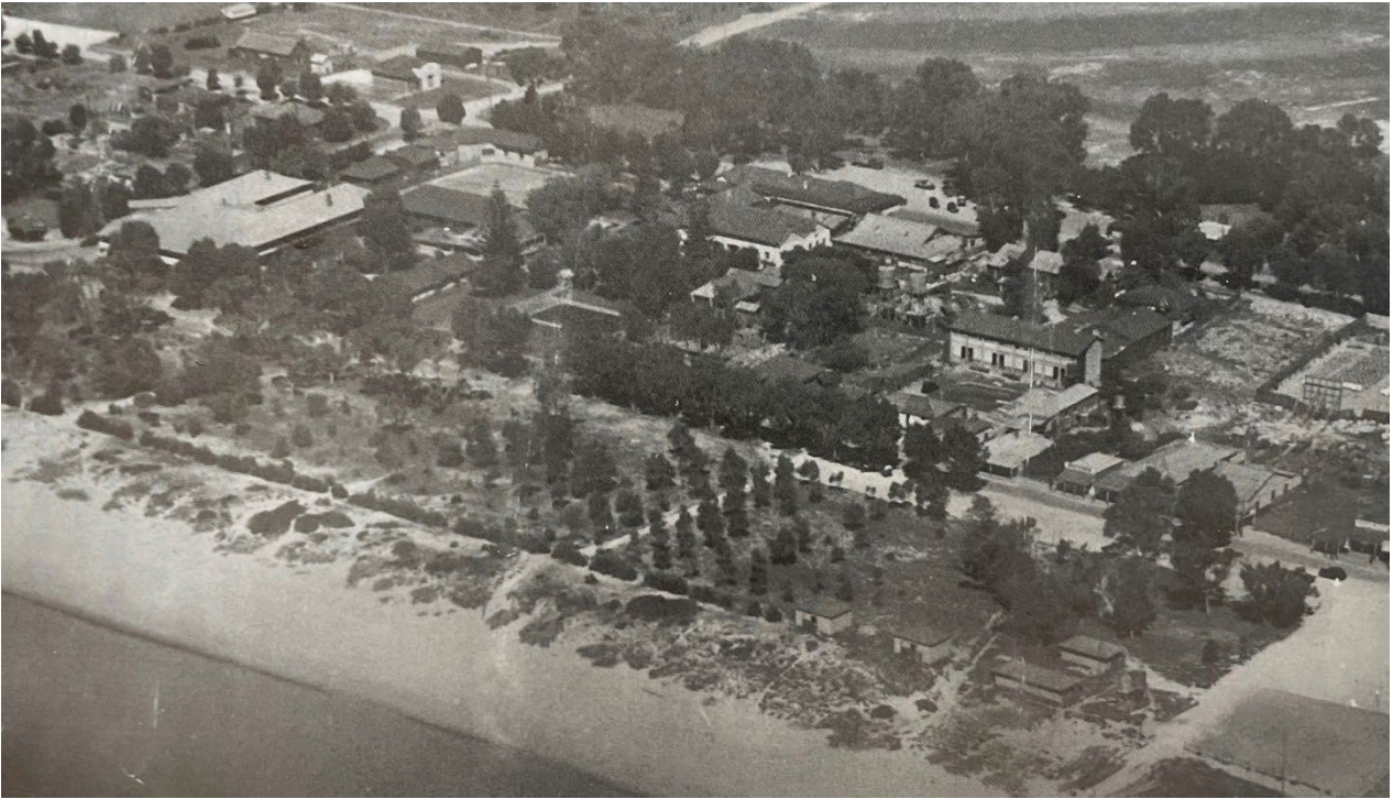
Aerial view late 1940s, Courtesy RDHS as reproduced in Draper & Kerford, Rockingham from Port 1872 to City 1988 , p. 152.
