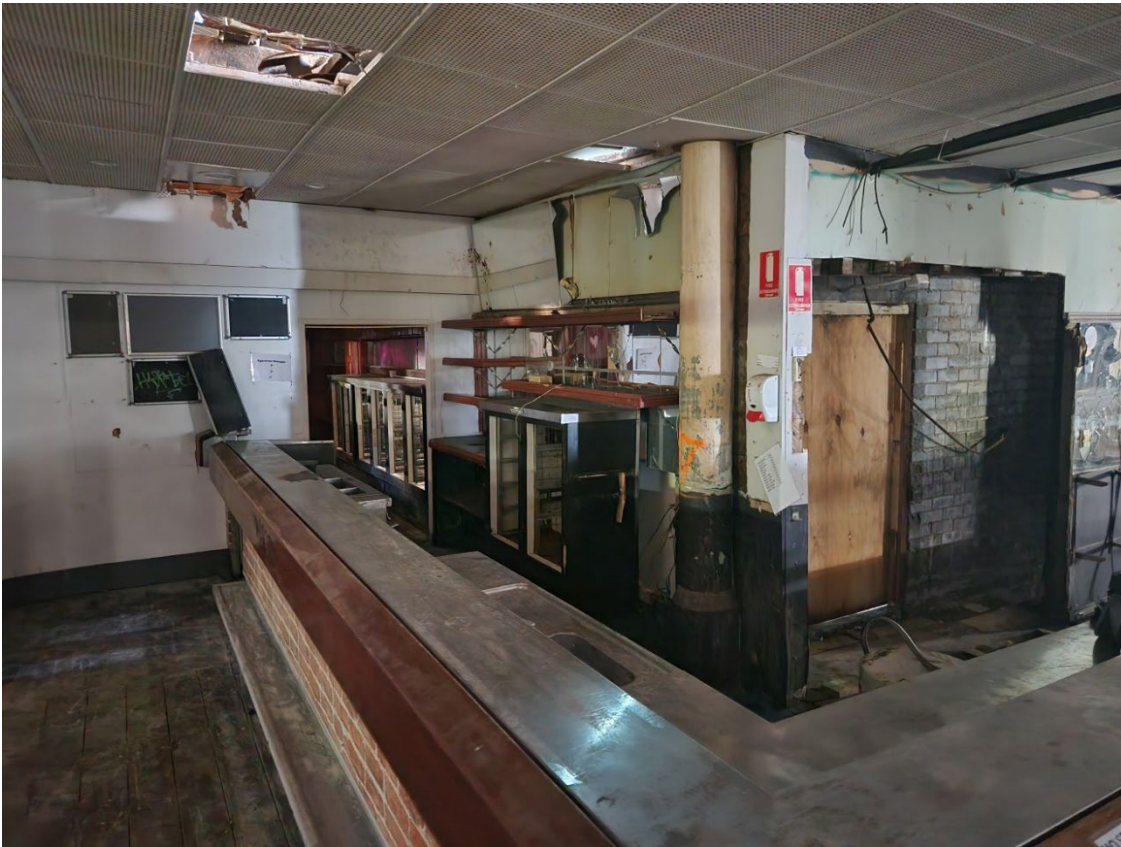
View 41 View of the counter from the Lounge
