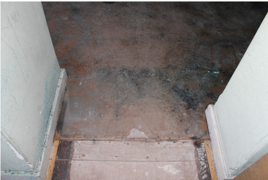
View 72 Floor threshold between the First Floor office and lounge
