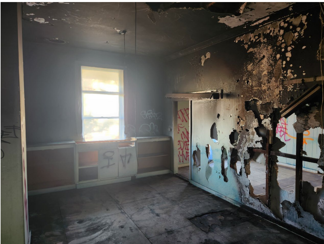
View 74 Cabinetry detail in the south wall of the Lounge
