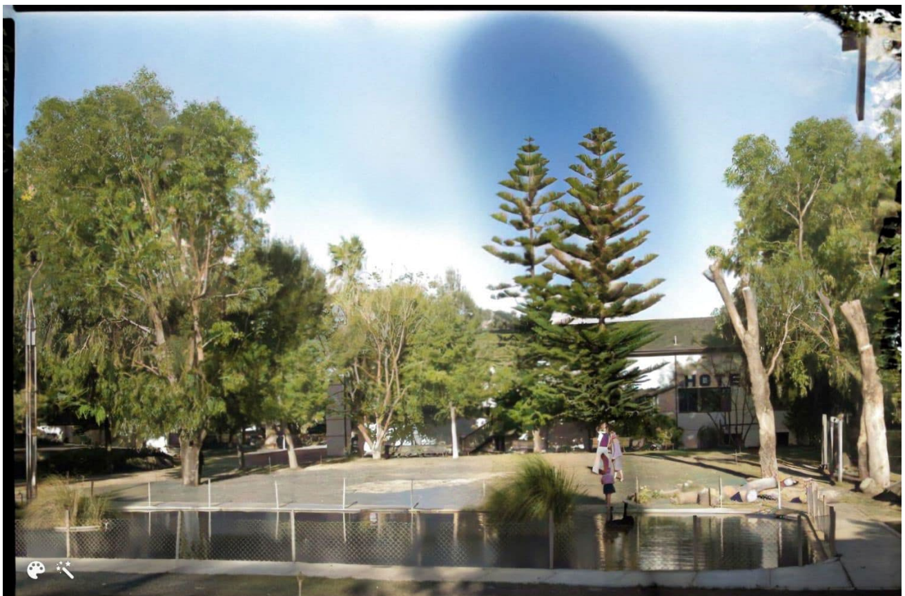
Figure 31 View of the northern elevation of the Rockingham Hotel, c1952 Courtesy Facebook History Rockingham | Kwinana
