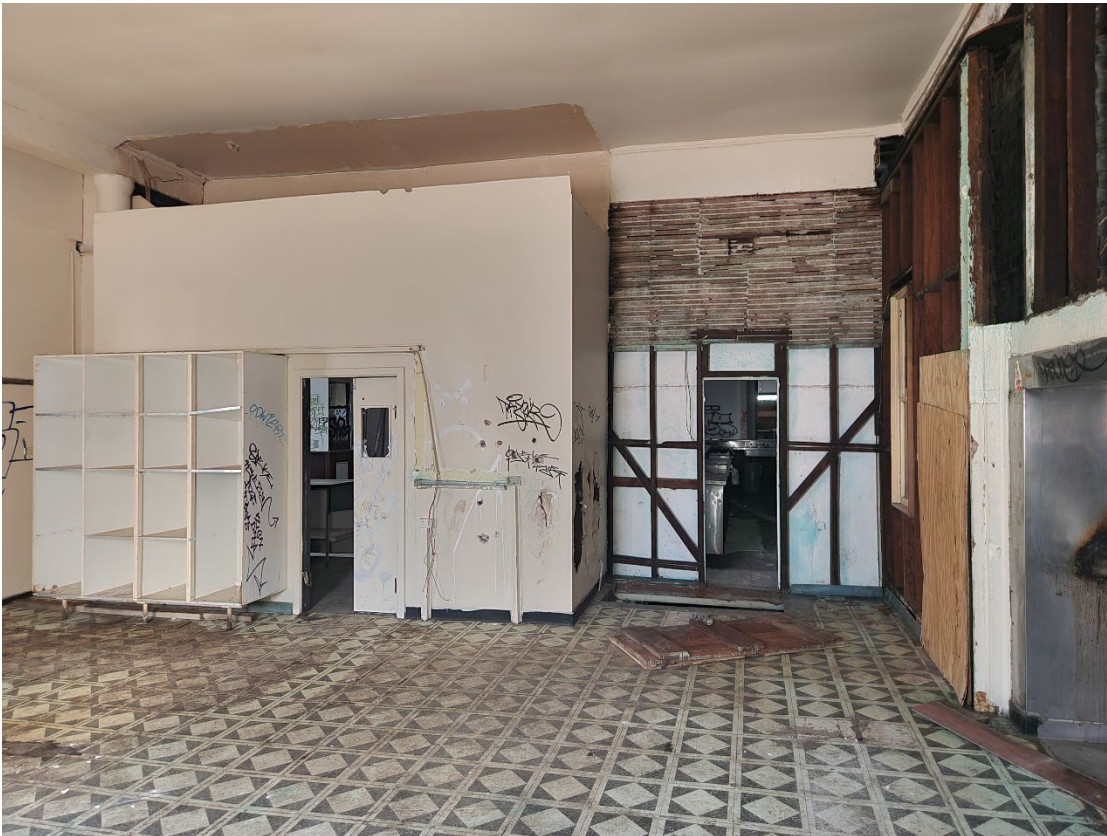
View 33 Doorways connecting the Kitchen and Dining Room
