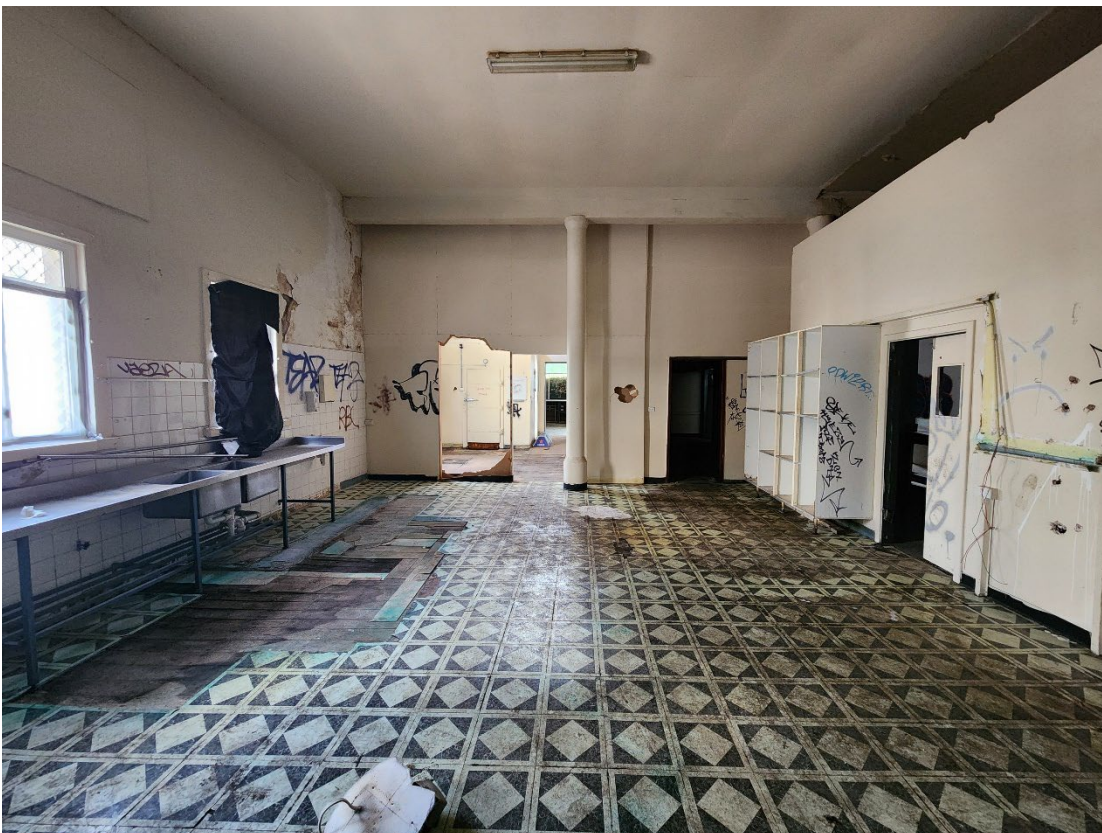
View 30 Vinyl flooring in the Kitchen with structural columns still extant
