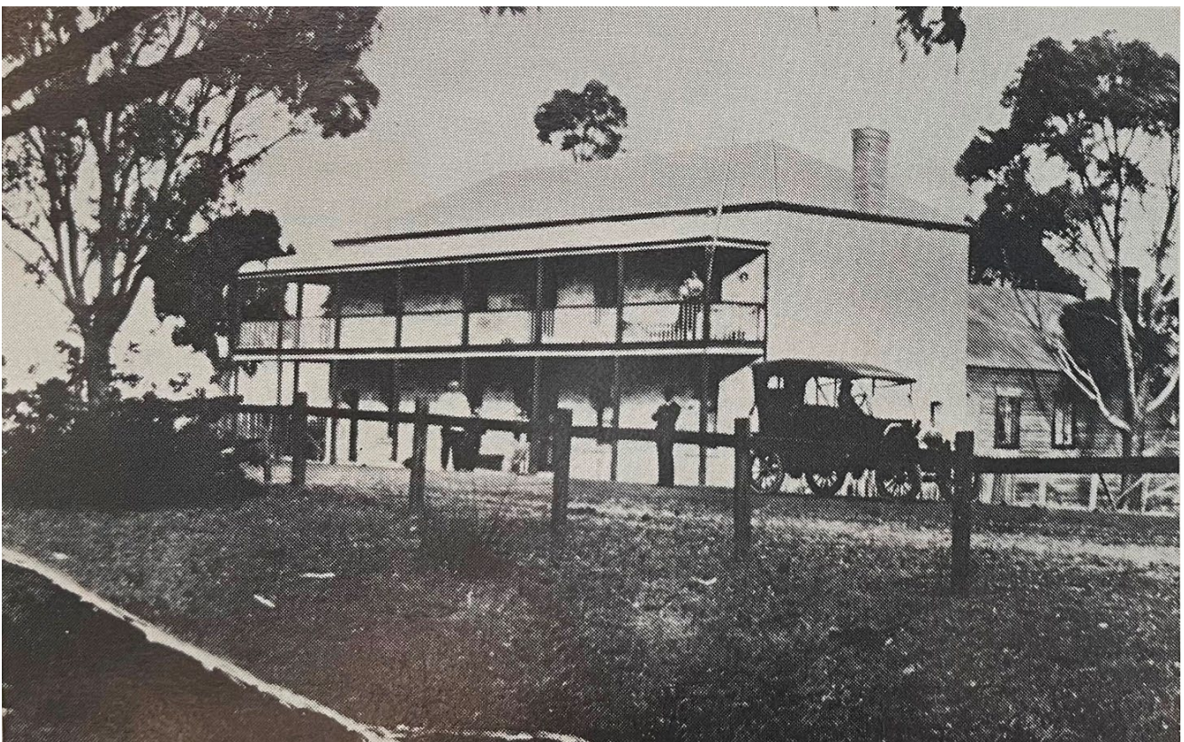
Figure 9 Port Hotel c1915 the verandah has been extended by one bay to the west to wrap around the western elevation Courtesy Rockingham Yesterday, Today & Tomorrow, p. 1
