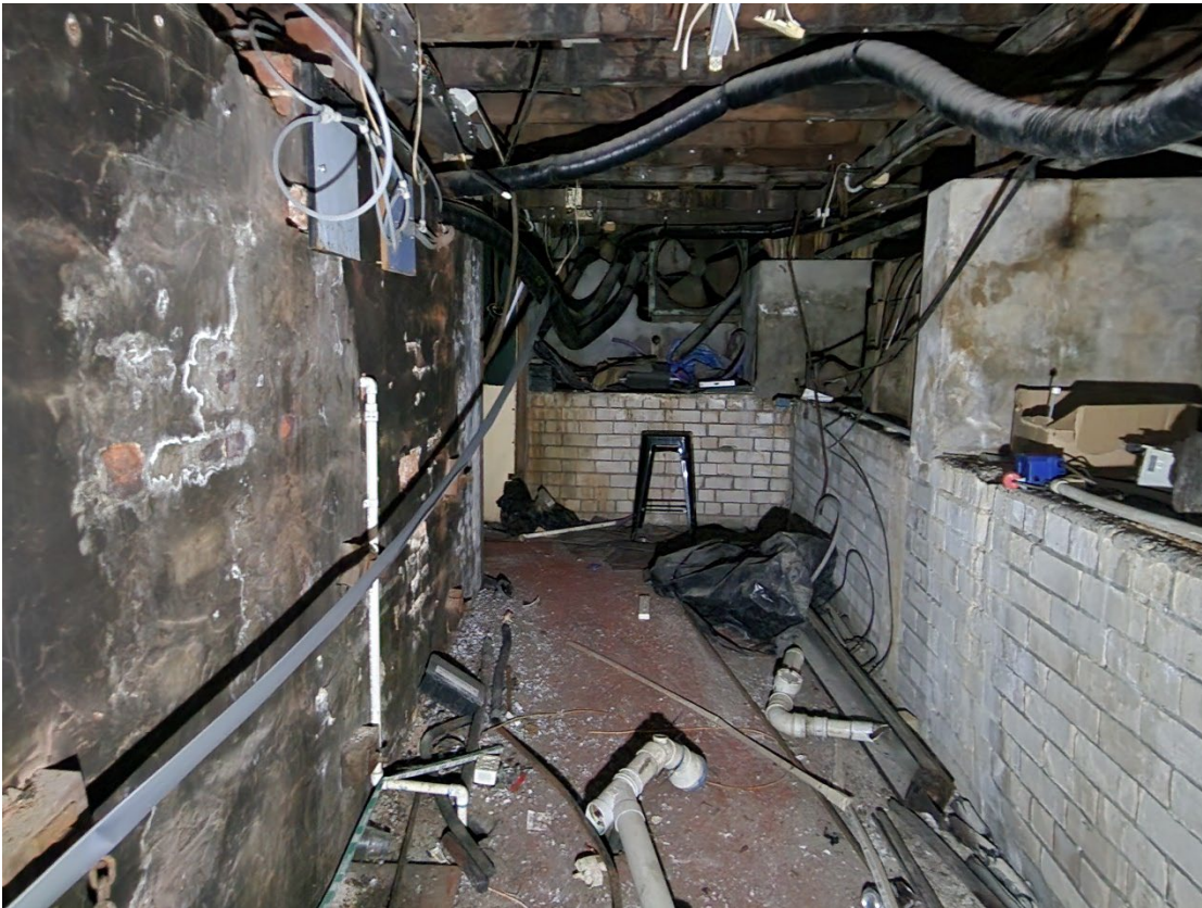
View 110 View in the basement
