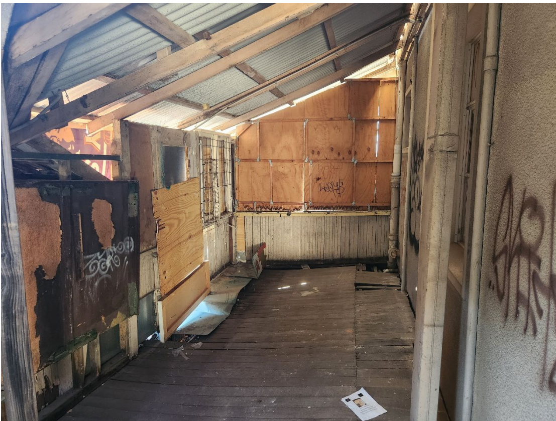
View 96 External area north of the Laundry in the First Floor
