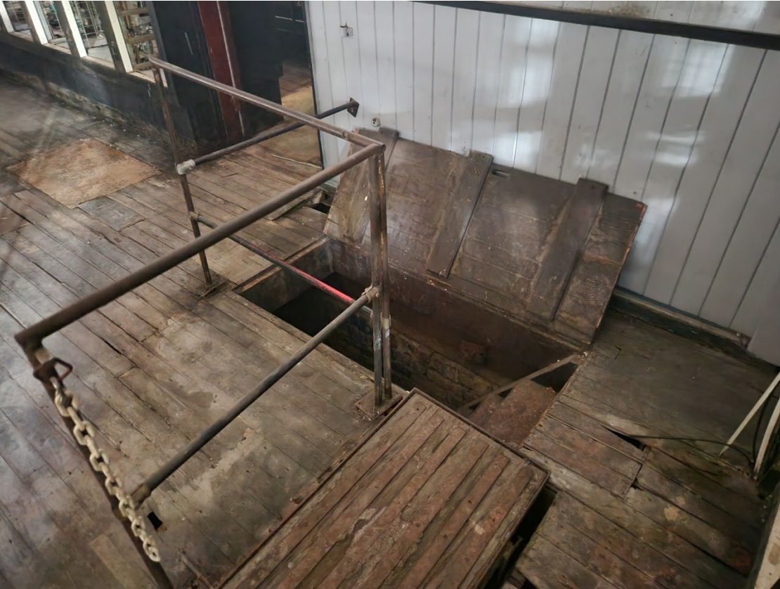
View 61 Trap door access to the basement from the Bar
