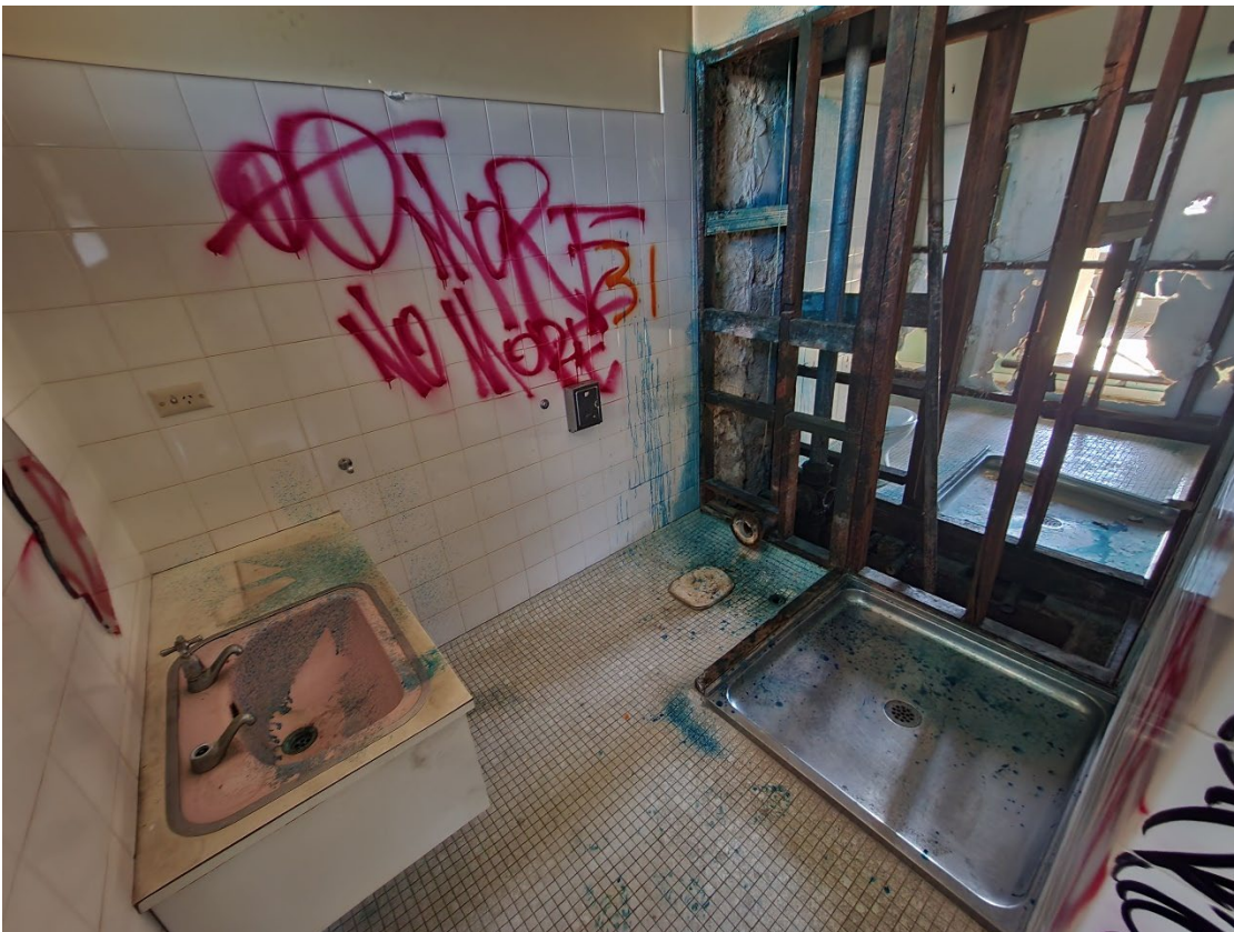
View 78 Room 1 bathroom interior with tiled floor and walls
