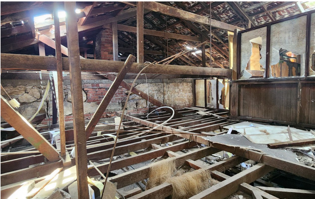
View 98 View of the roof space above the over Saloon
