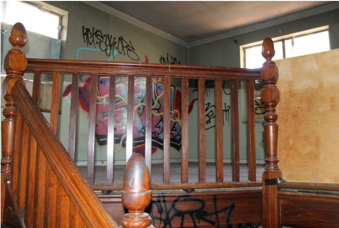
View 69 Detail of timber balustrade in the upper floor
