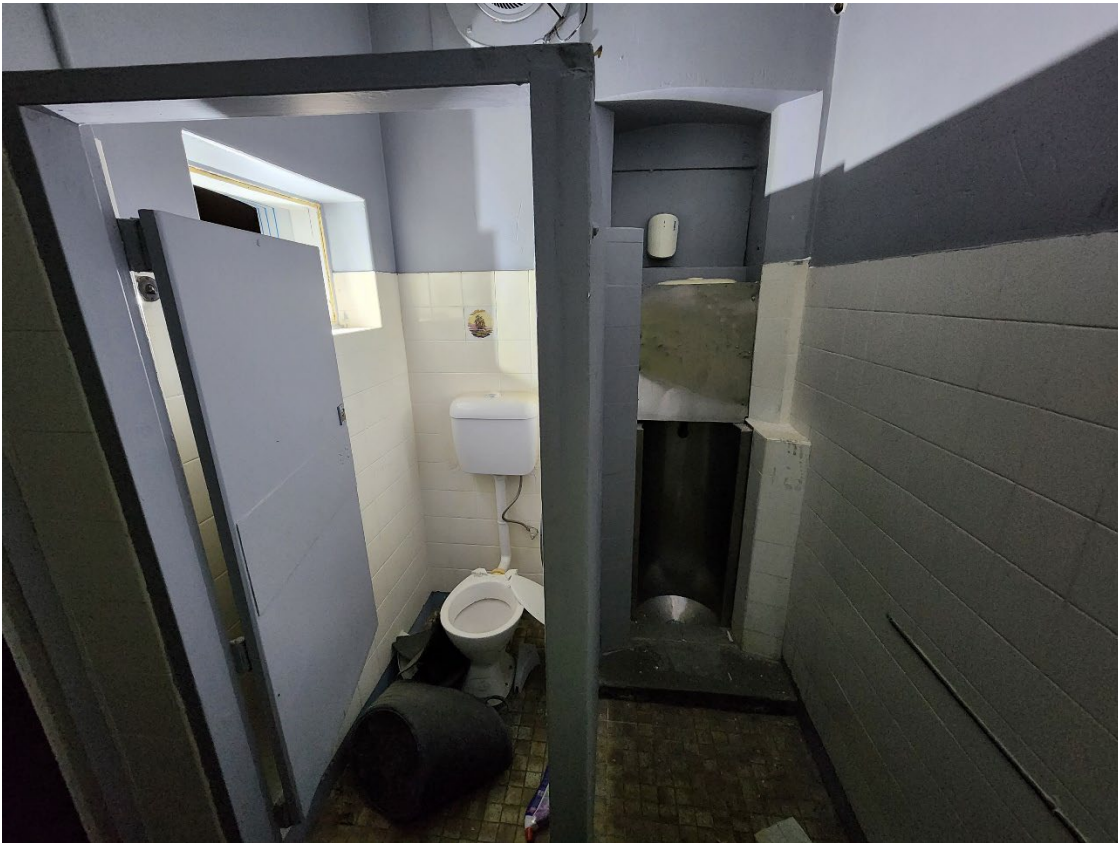
View 51 Fitout of male toilet
