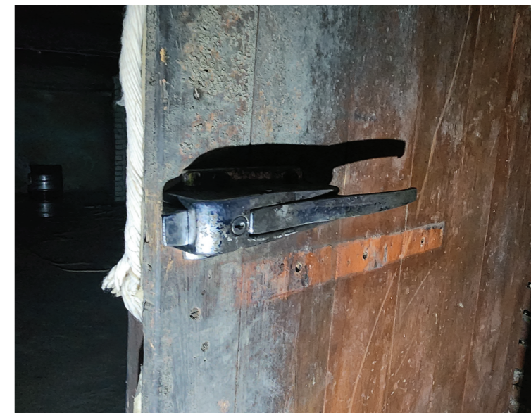
DOOR HANDLE TO STORE ROOM AT BASEMENT
