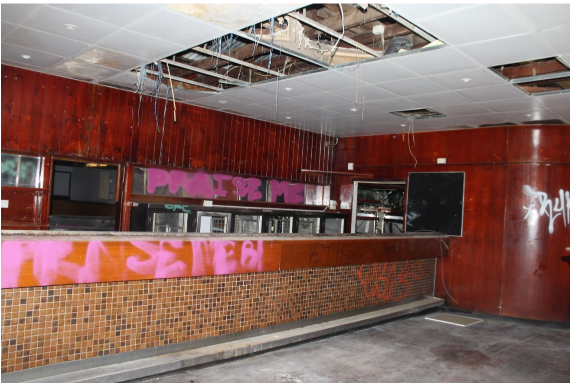
View 54 Counter in the Saloon and timber panelling and boards around the walls and bulkheads
