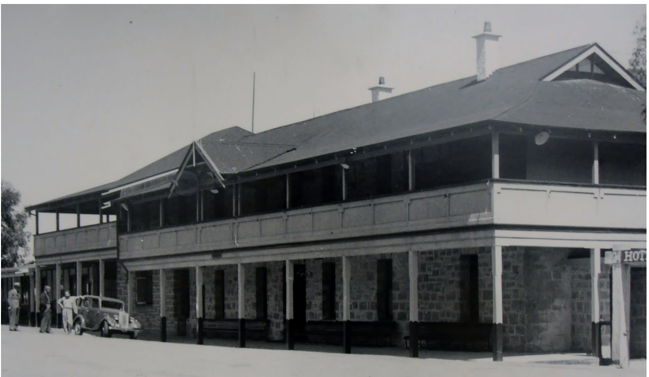
Figure 23 Hotel Rockingham, c1938 showing the addition on the western elevation at a higher level Courtesy Facebook History Rockingham | Kwinana
