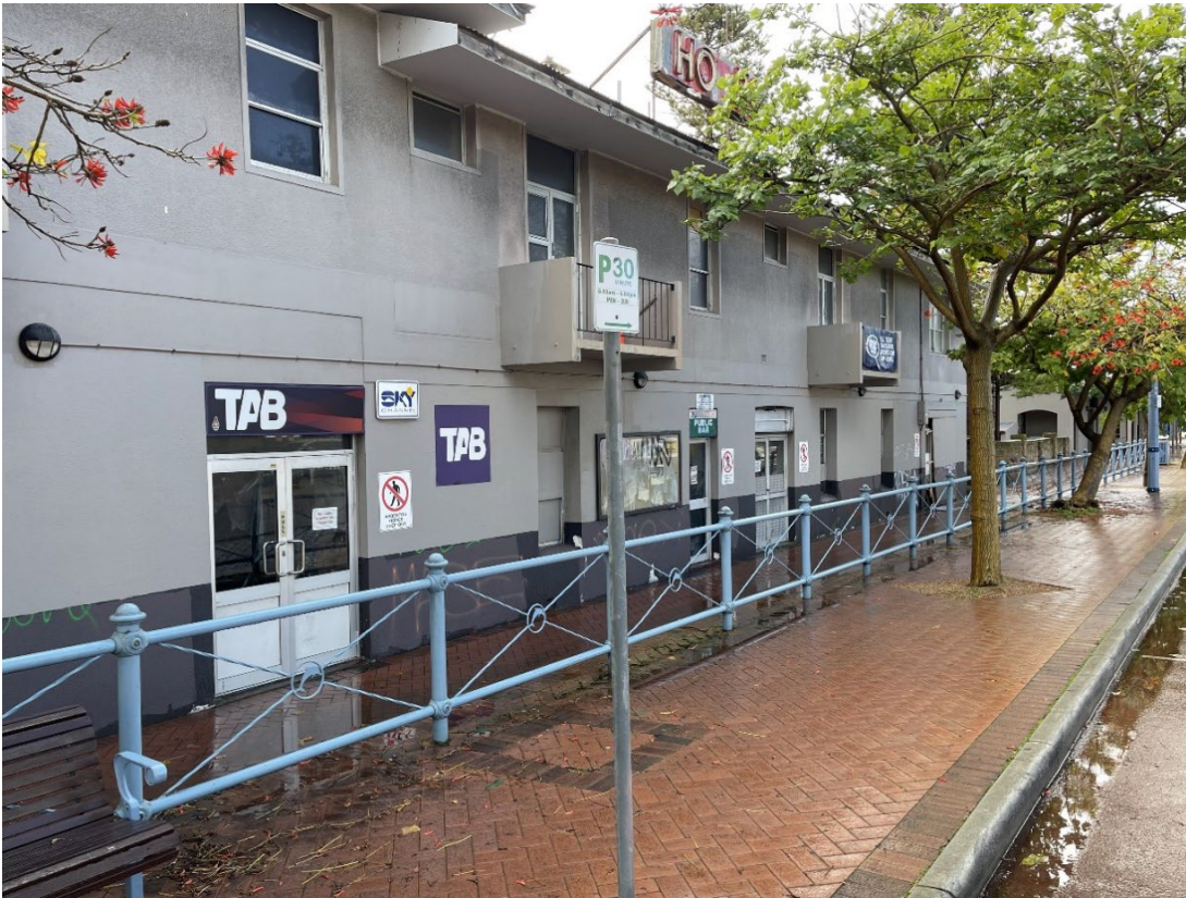
View 9 Balconies on the southern side of Rockingham Hotel facing Kent Street Courtesy Emirge, June 2023
