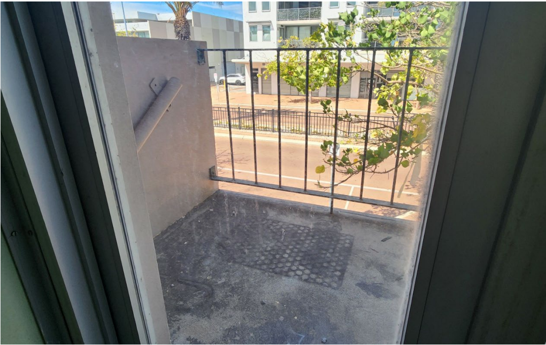
View 87 View of the balcony off Room 5
