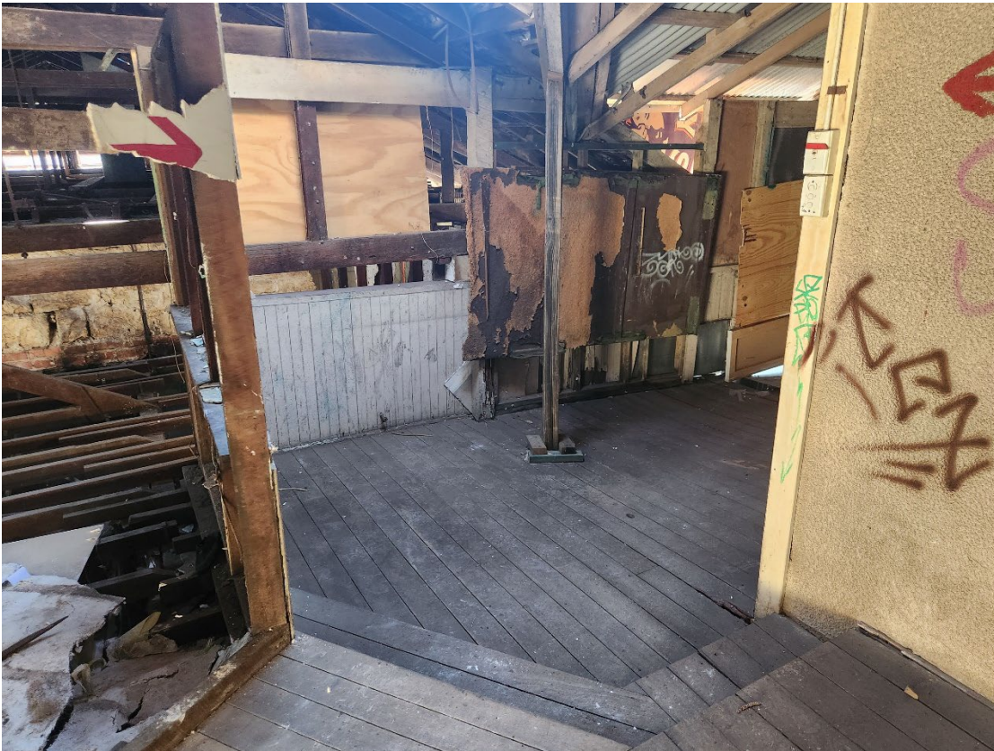
View 95 Timber steps down into the lower section of the verandah
