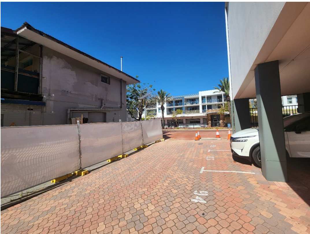
View 8 Western side of the building from the neighbouring accessway
