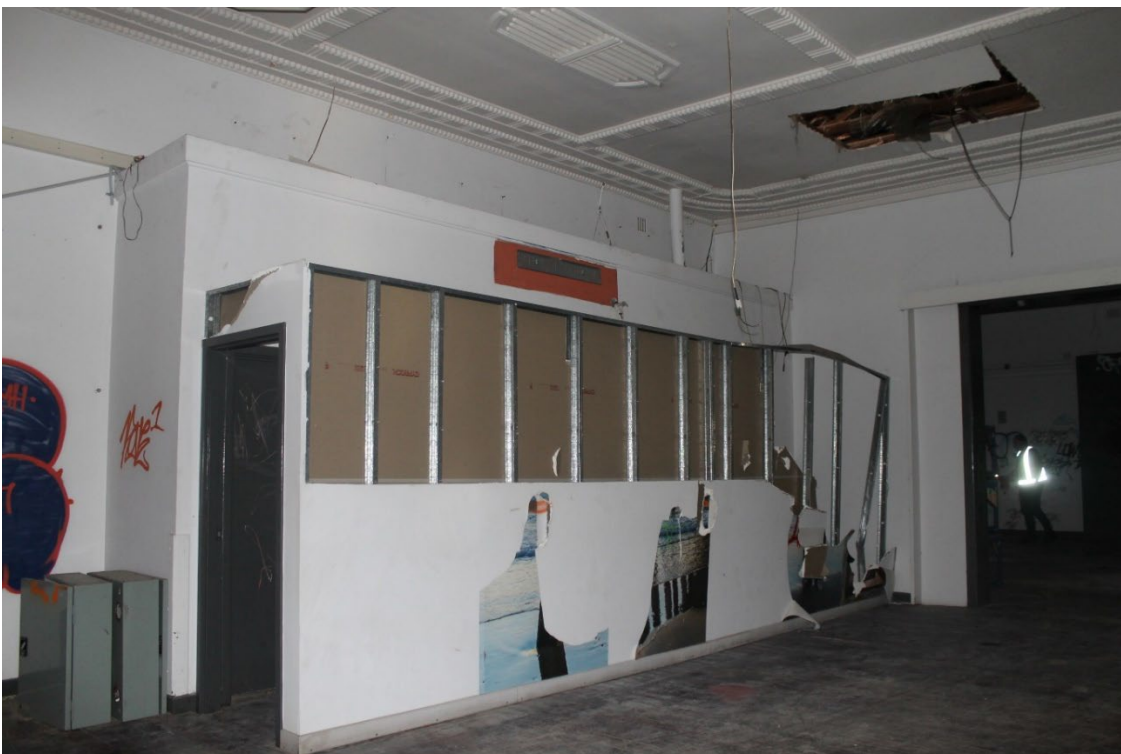
View 42 Access to the toilets from the Dining Room area
