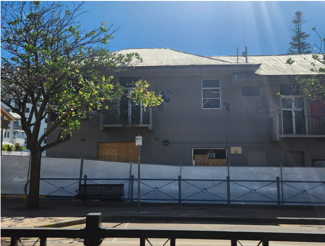
View 19 View of the southern corner facing Kent Street
