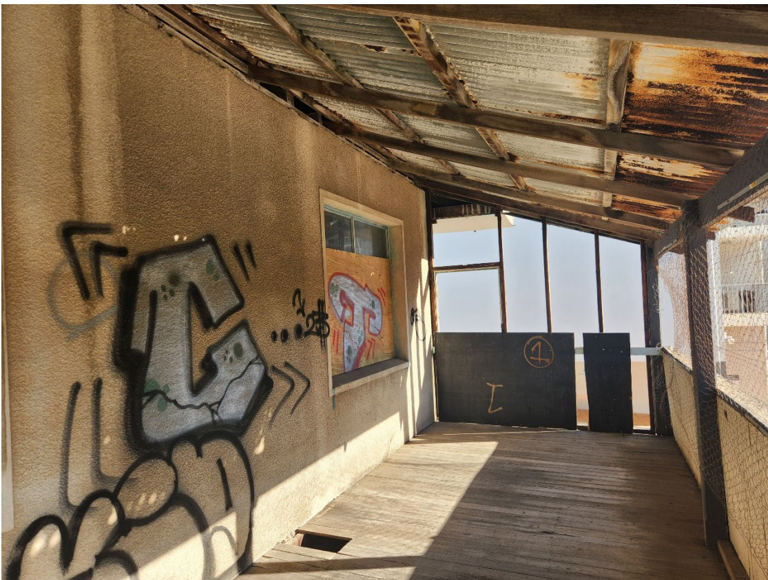
View 92 Looking towards the west of the verandah
