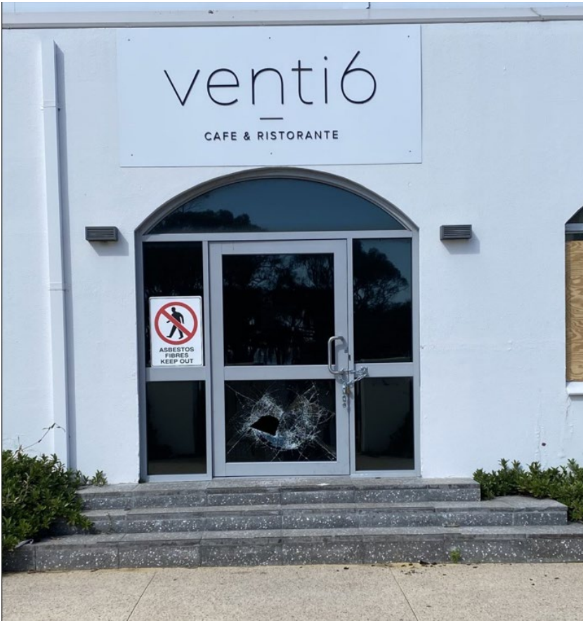
View 15 Raised entry connecting the Beer Garden and Function Room inside Courtesy Emirge, June 2023
