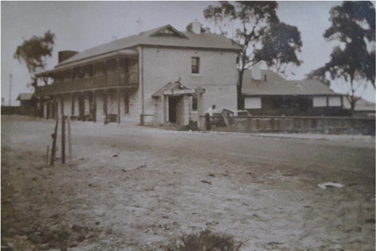
Rockingham Hotel, c1922 showing the addition at the eastern end of the elevation and the enlarged single storey portion of the hotel. Courtesy Facebook History Rockingham I Kwinana.
