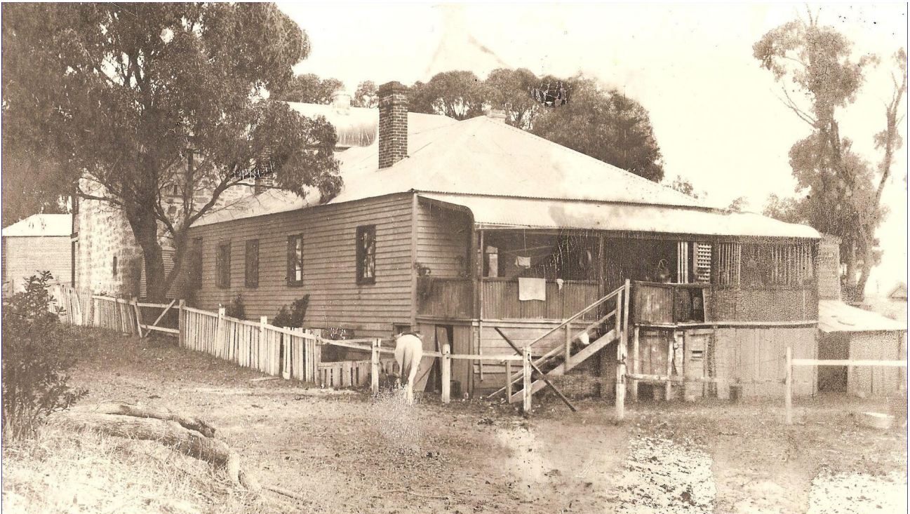
Figure 6 Port Hotel, 1898, viewed from the foreshore side showing the original simple weatherboard construction and the stone addition to the rear on Kent Street
