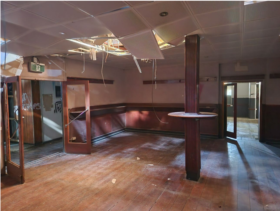
View 53 Saloon interior with 160mm wide timber floorboards and timber dado
