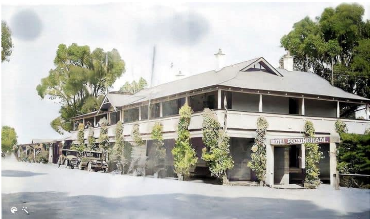
Rockingham Hotel, c1935 at the opening of the electric light in Rockingham. Courtesy History of Rockingham / Kwinana Facebook page, colourised by My Heritage.
