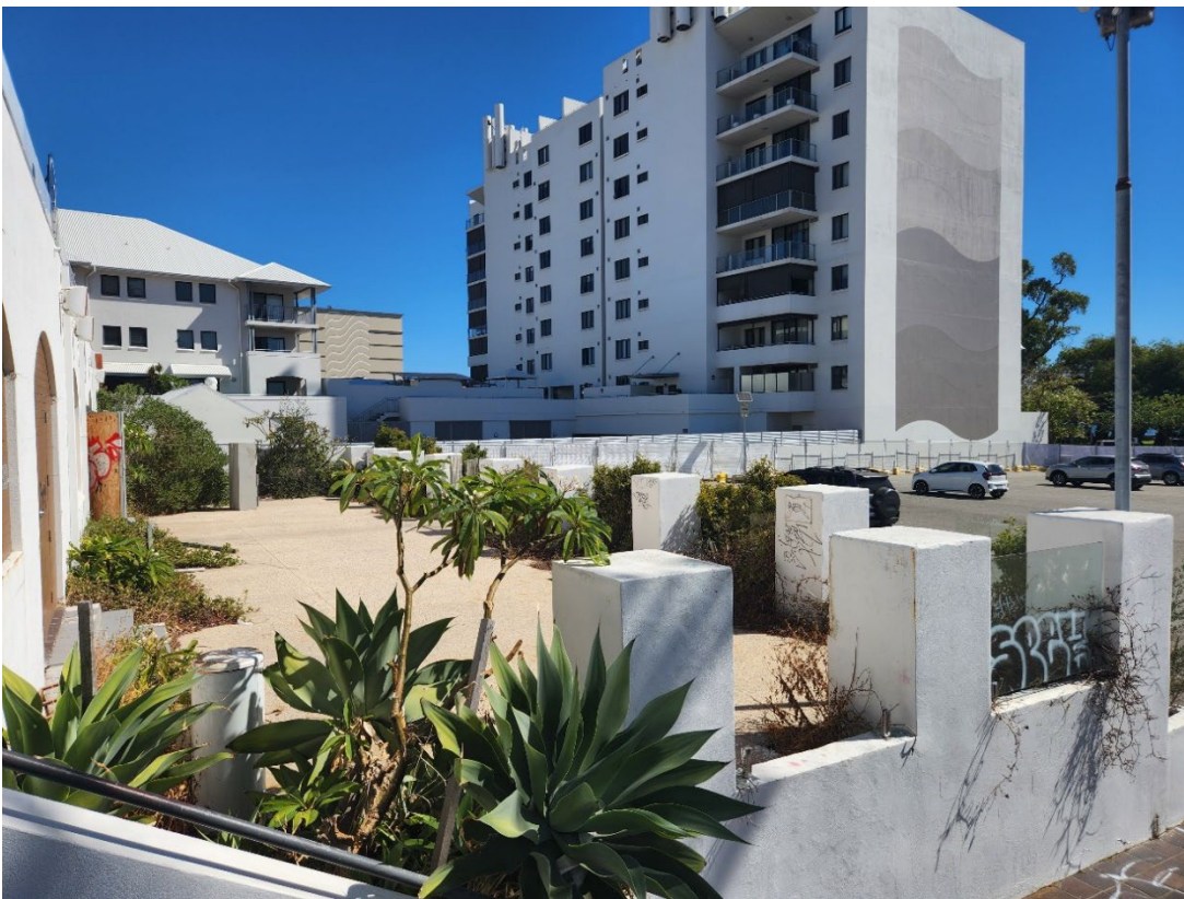
View 4 View of the beer garden and carpark over from the entry staircase
