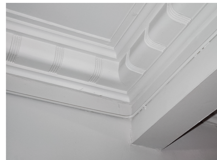
DETAIL OF CORNICE IN POOL ROOM
