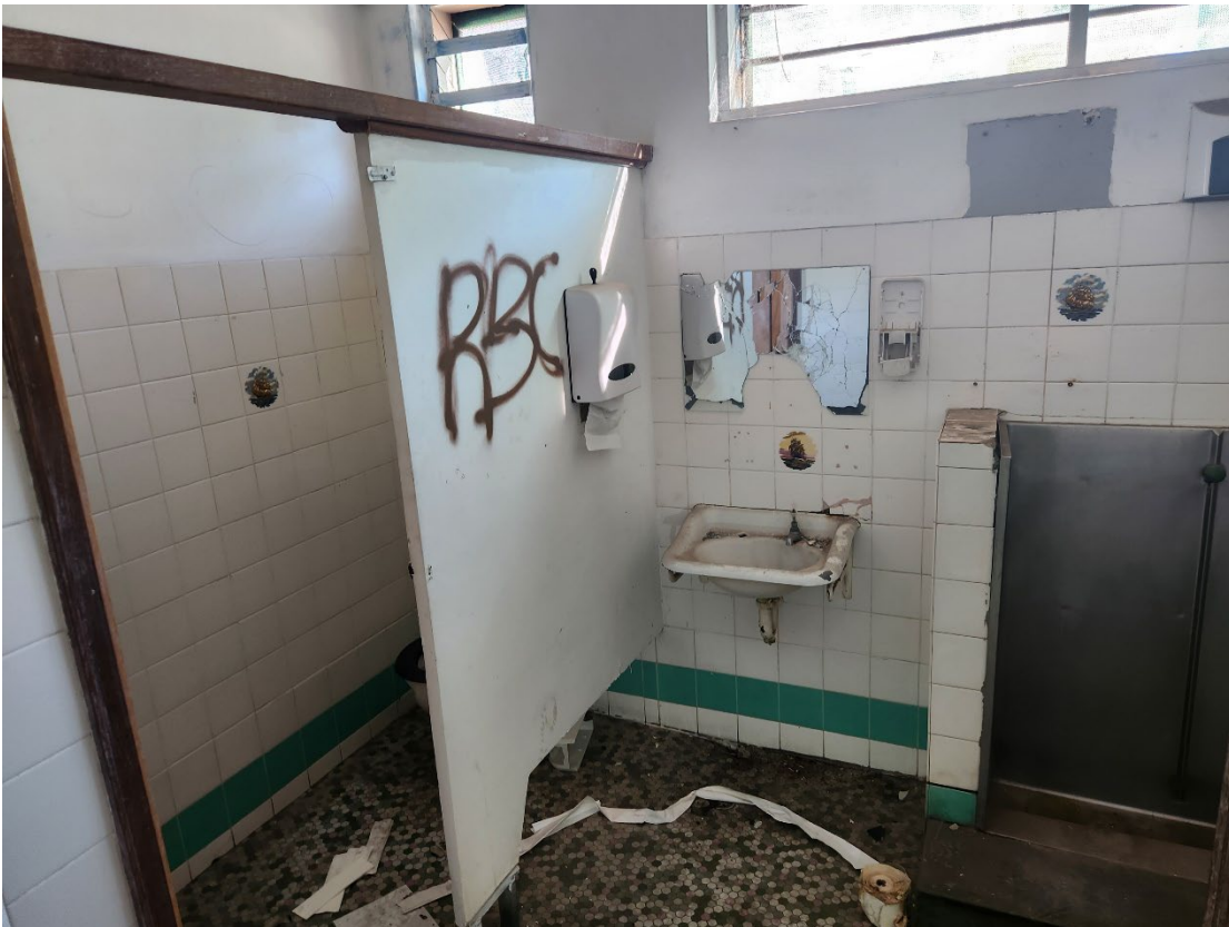
View 62 Interior of the toilets off the Bar
