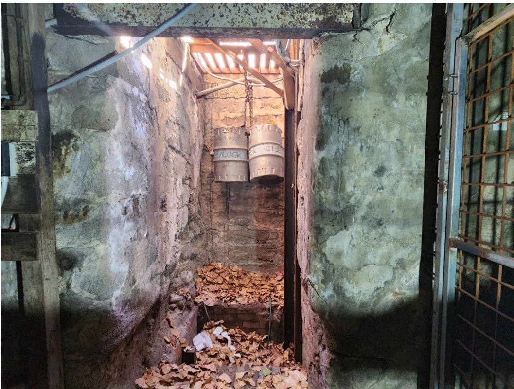
View 104 Area open to the outside
