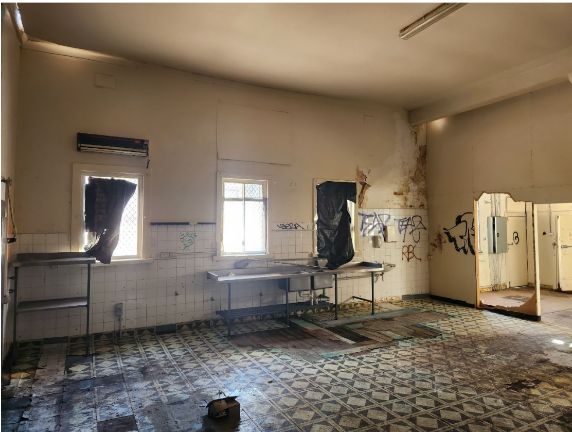
View 32 Extant bench and plumbing fixtures in the Kitchen
