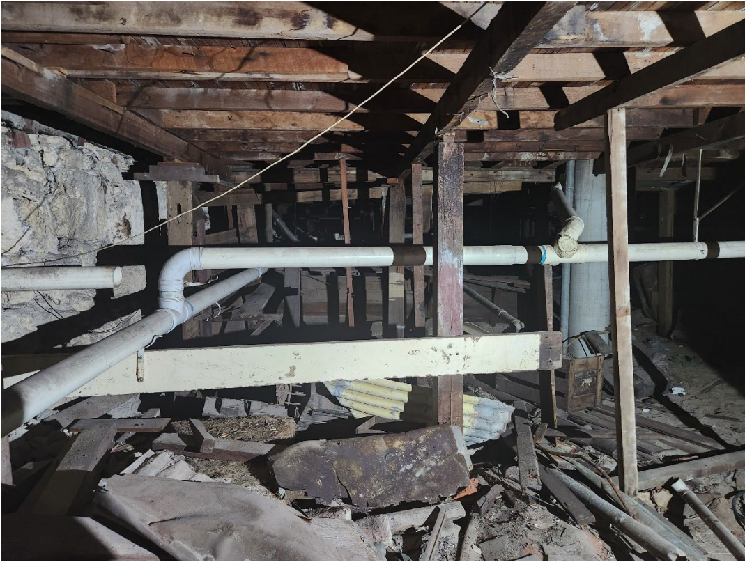
View 113 Service pipes in the basement
