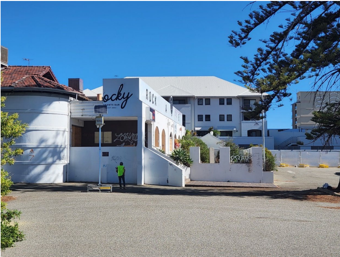
View 3 Northeast corner of the building
