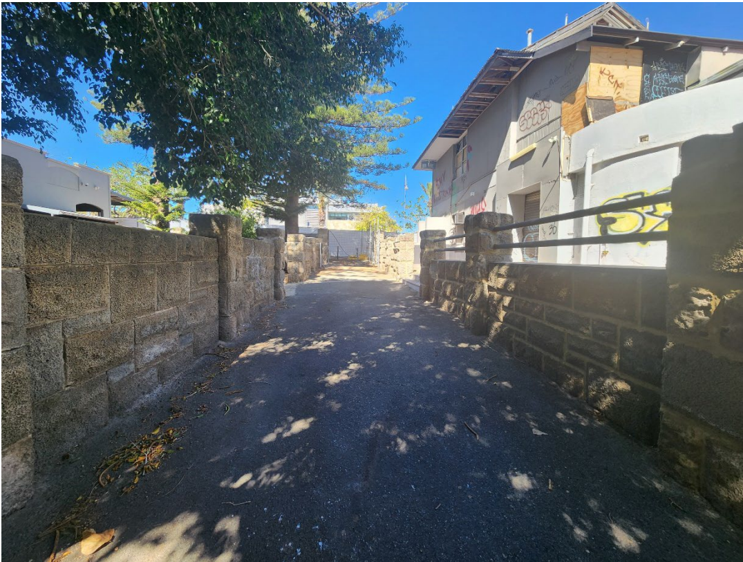
View 5 Vuggy limestone walls lining the accessway to Kent Street
