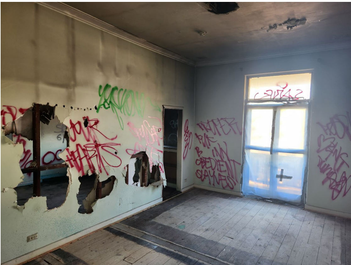
View 76 Room 1 interior
