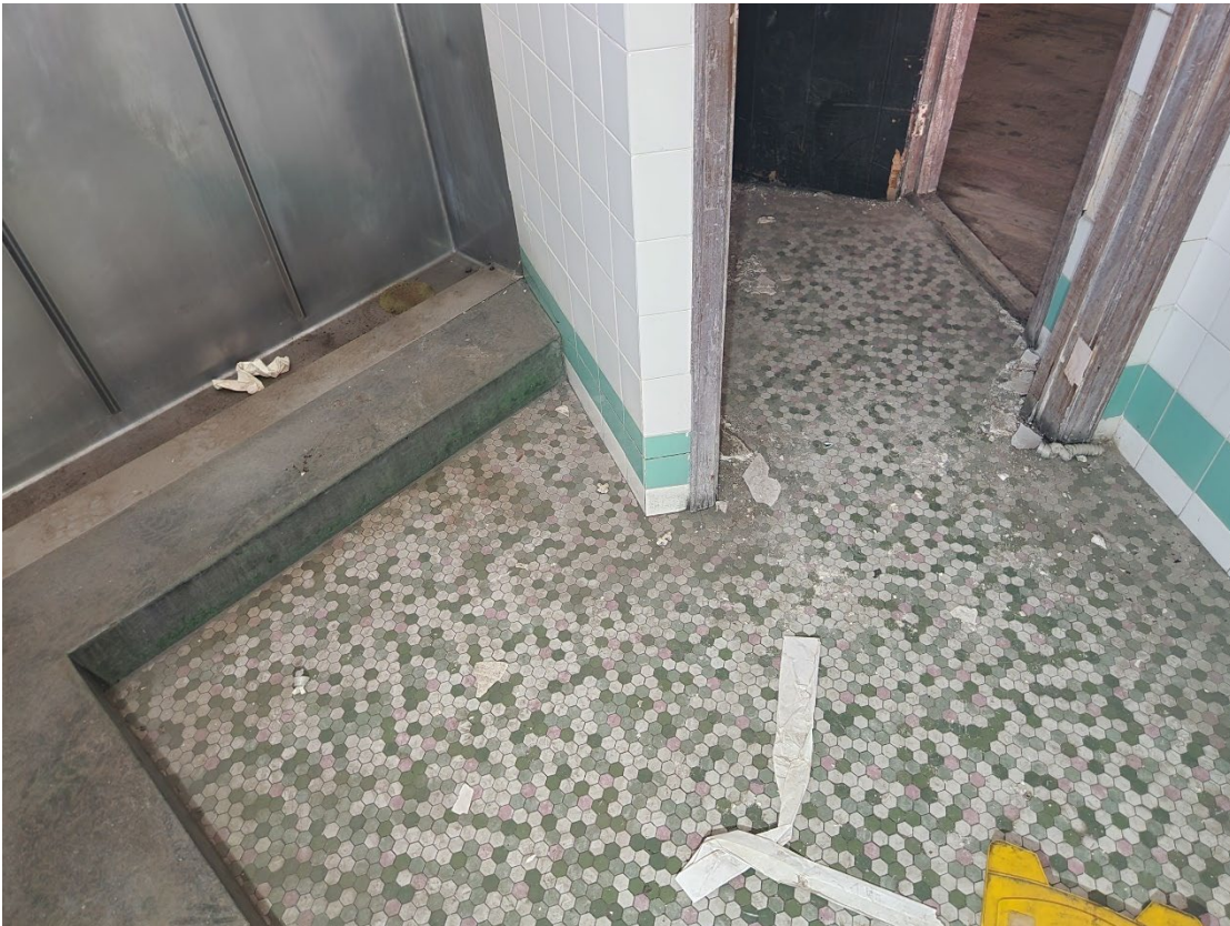
View 63 Detail of mosaic tile flooring in the toilets off the Bar
