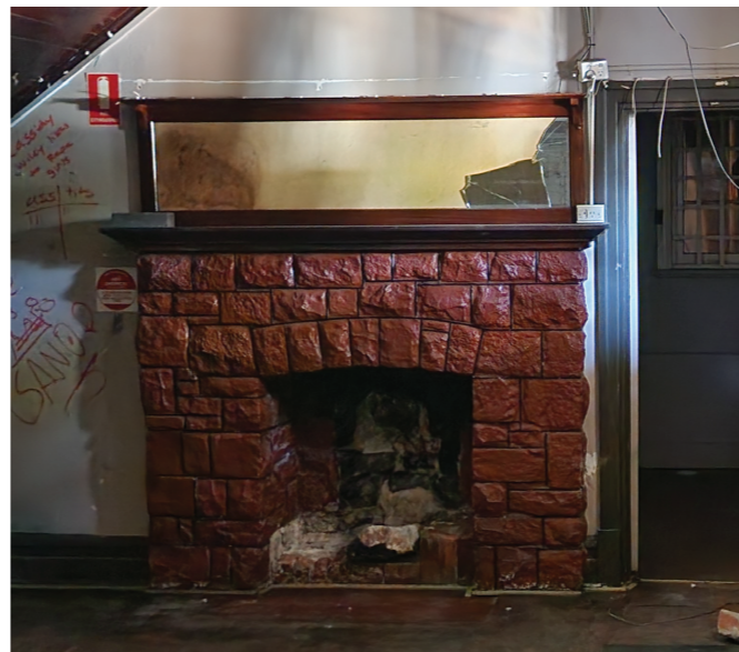
FIREPLACE AT GROUND FLOOR OFFICE
