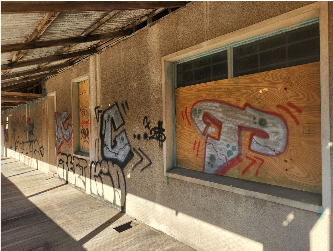
View 93 Openings in the First Floor external wall facing the
