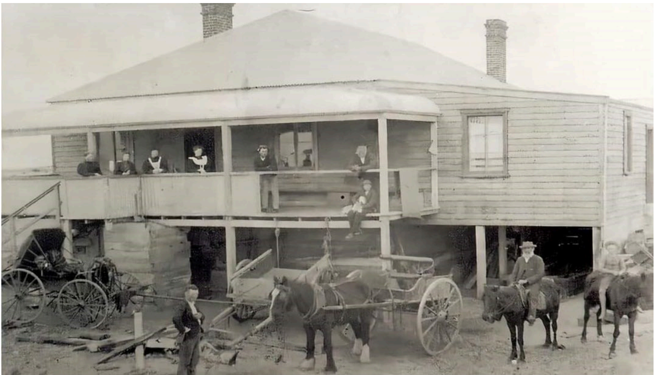
Figure 5 Port Hotel, c1890s, a simple weatherboard construction by James Bell Snr Courtesy Facebook History Rockingham | Kwinana
