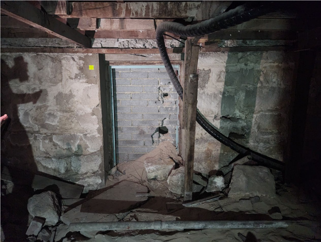
View 113 Brick infill in opening in the basement
