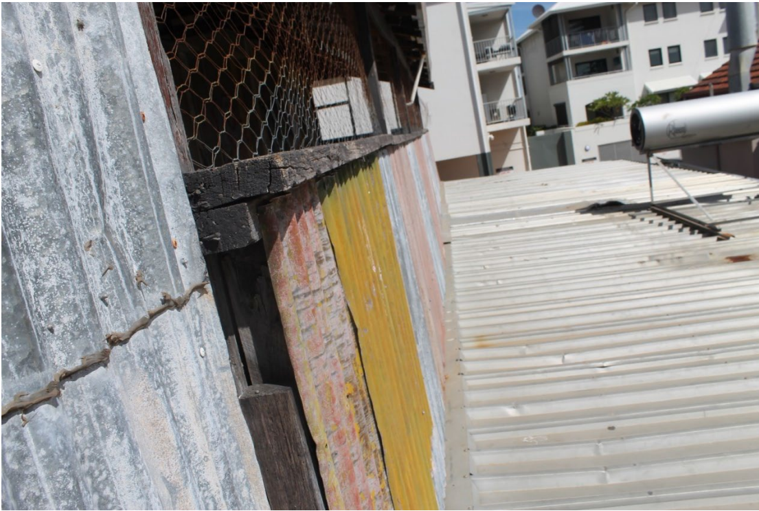
View 101 Timber structure and metal cladding of the verandah
