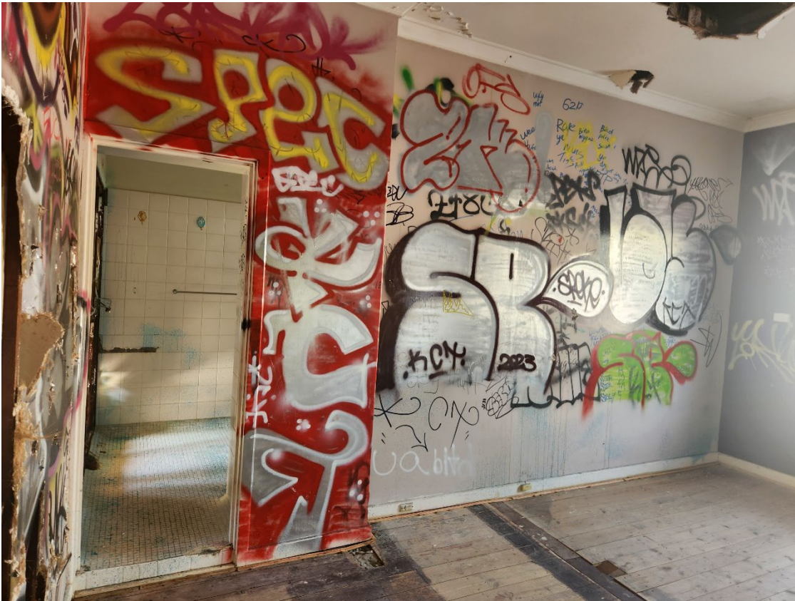
View 79 View of stepped access into Room 2 bathroom
