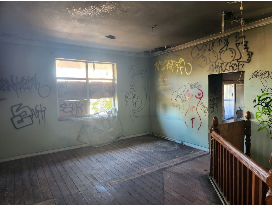
View 70 First Floor Office showing the access into the Lounge
