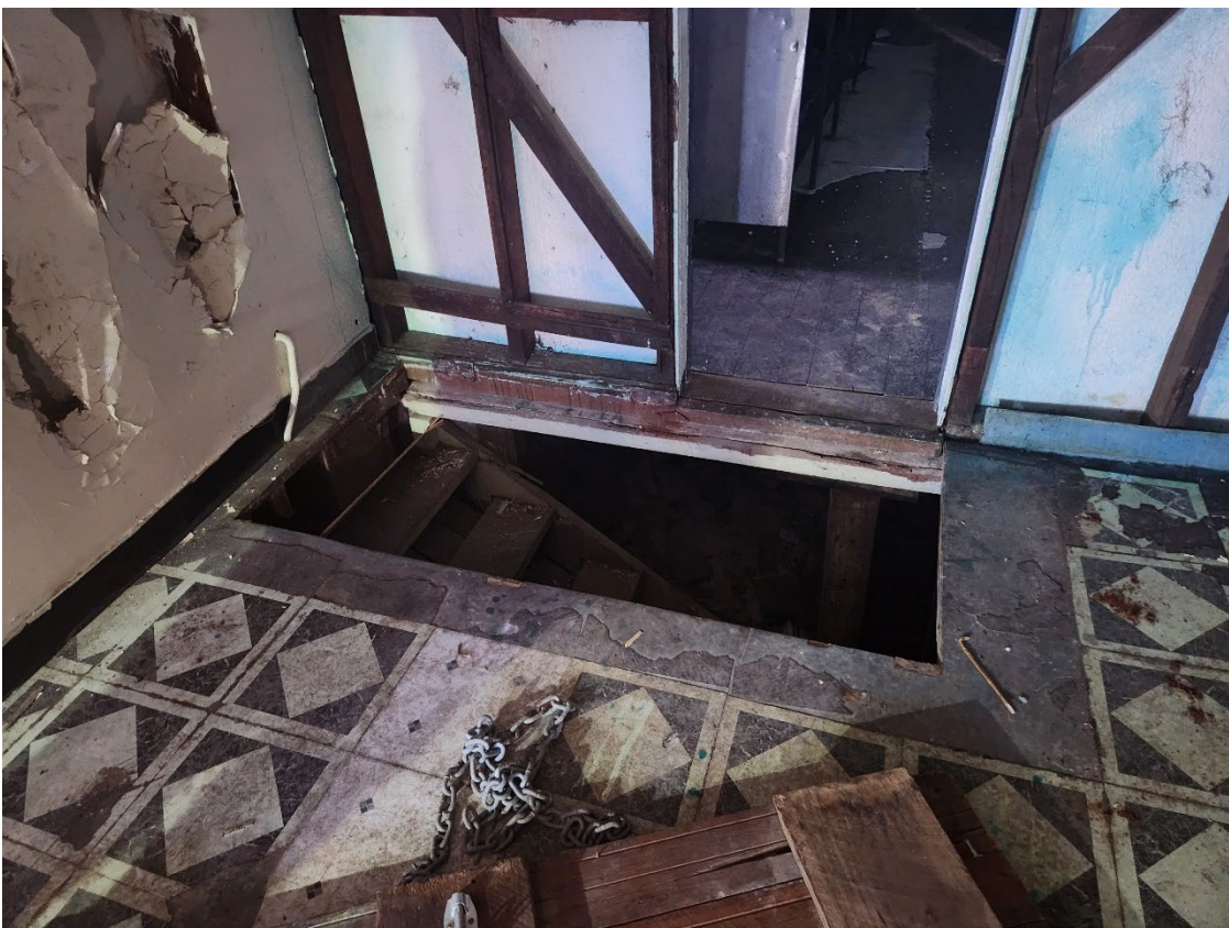
View 34 Trap door access to the Basement from the Kitchen floor
