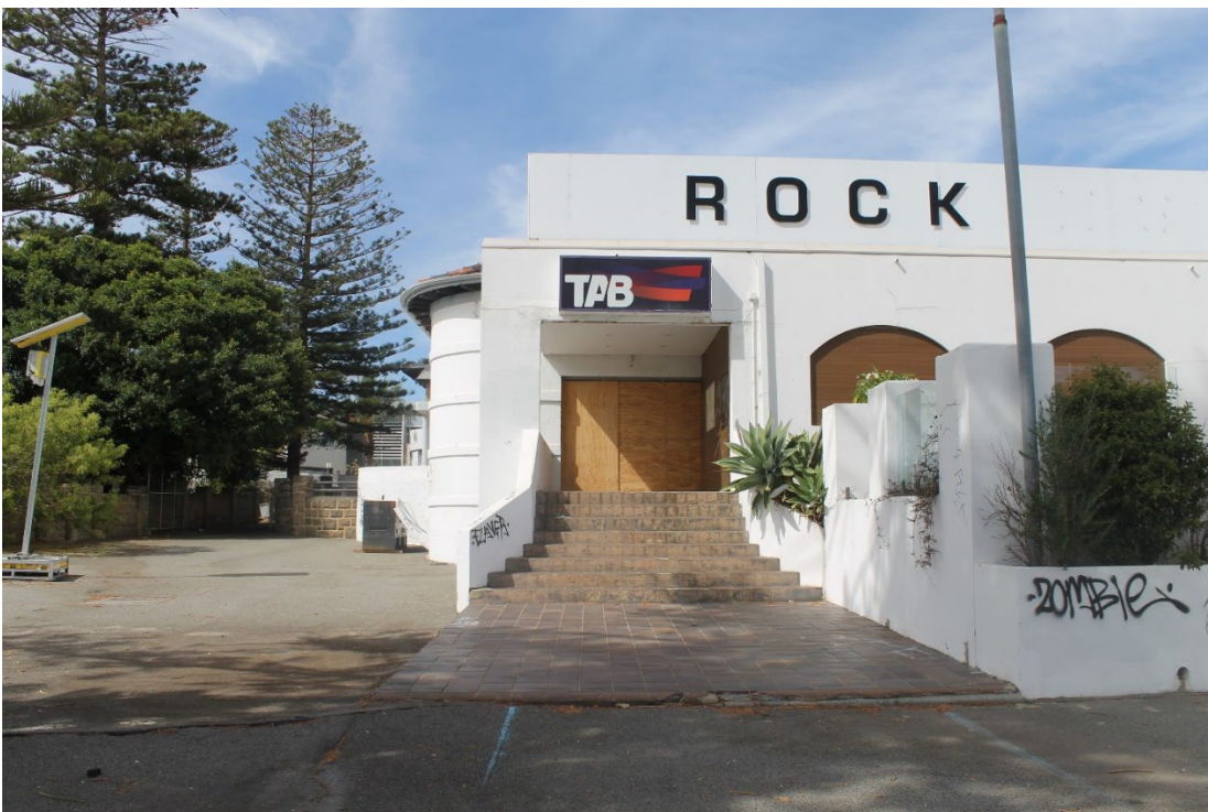
View 12 Main entry staircase accessed from carpark
