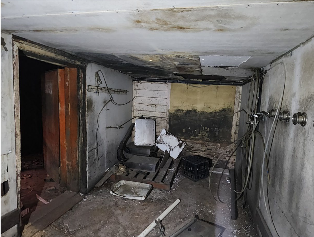
View 103 Inside one of the lockable rooms in the basement
