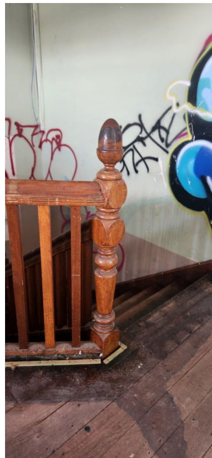
View 68 Detail of timber staircase (left) and newel post (right) leading to the upper floor
