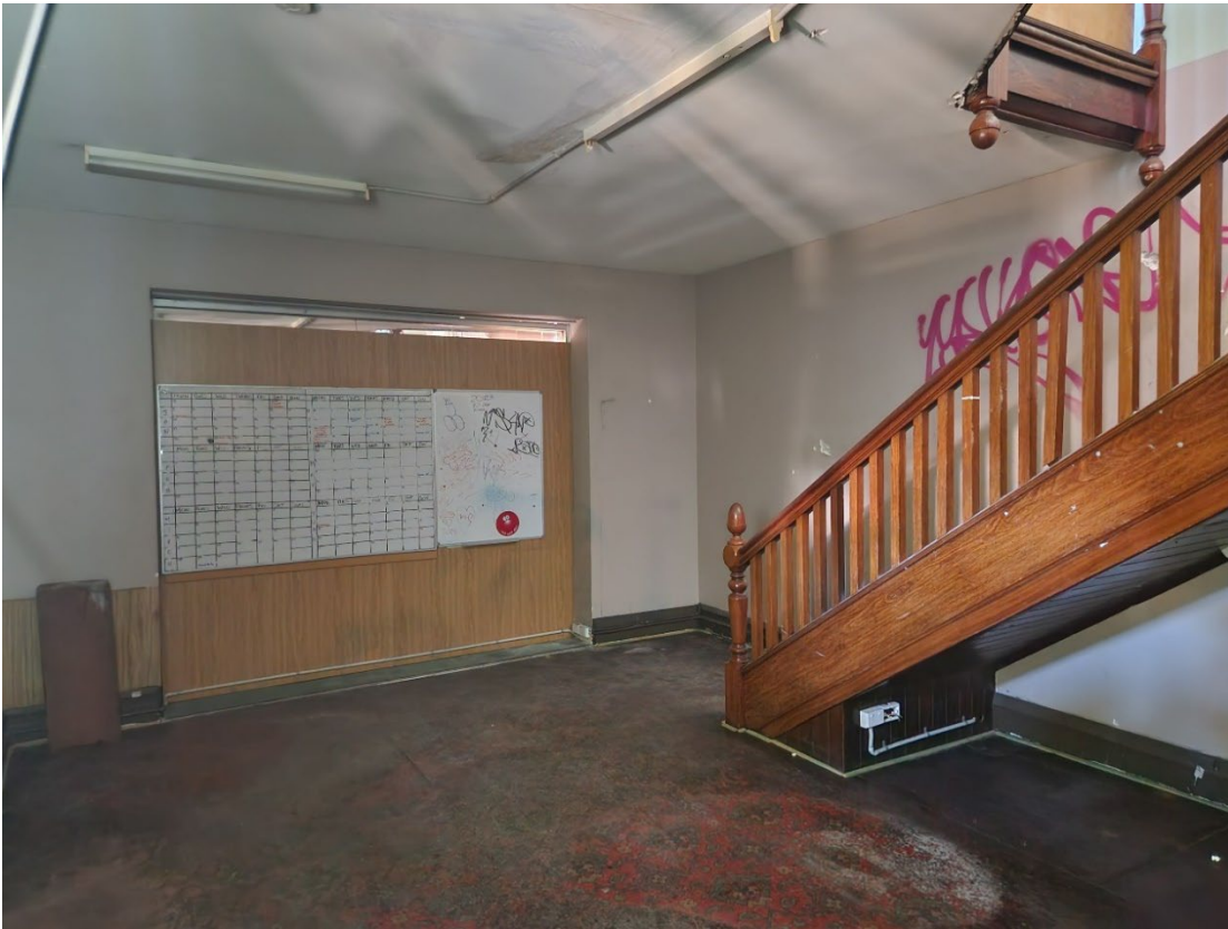
View 67 Stair access to the upper floor from the Office
