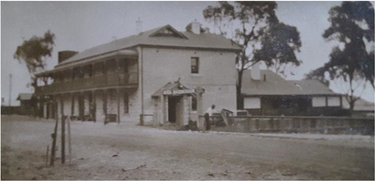
Figure 11 Rockingham Hotel, c1922 showing the addition at the eastern end of the elevation which created a new entrance on the east elevation, extension toward the original single storey building which included a small gable in the roof. The single storey portion of the hotel was substantially rebuilt and features new verandahs Courtesy Facebook History Rockingham I Kwinana
