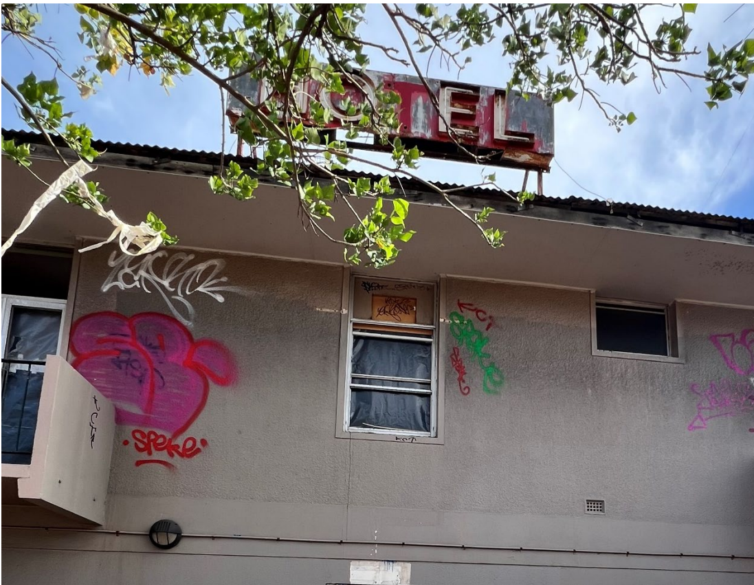
View 22 Wide eaves of the upper storey with timber fascia exposed and 'HOTEL' neon sign still extant
