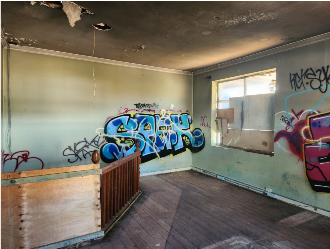
View 71 First Floor Office with timber floor boards
