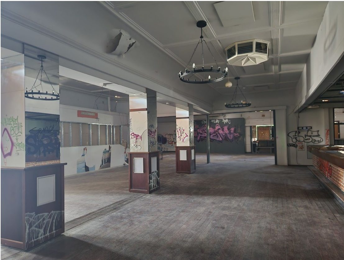
View 37 View of the Dining Room with timber floorboards
