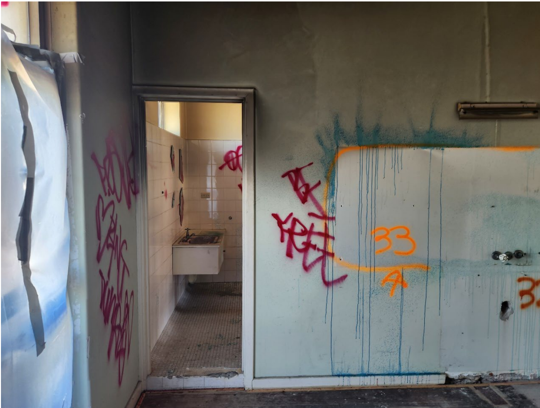
View 77 Stepped access up to the bathroom in Room 1
