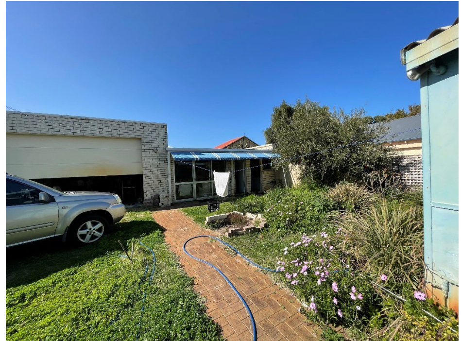
Figure 12: Brick garage and studio
