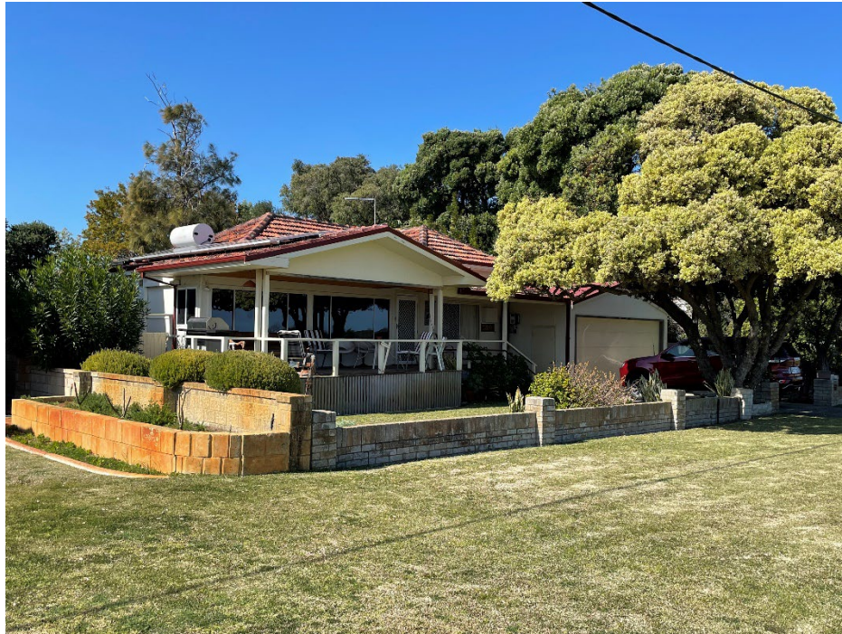
Figure 27: 116 Arcadia Drive included on the LHS in good condition
