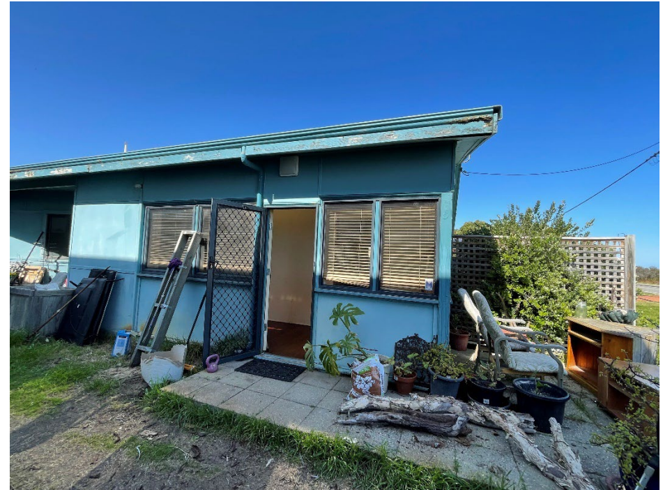
Figure 6: Main entrance to north elevation
