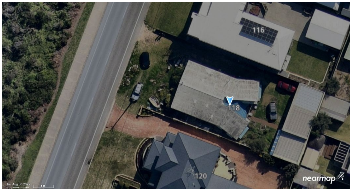
Figure 3: Aerial view of no. 118 Arcadia Drive, Shoalwater Courtesy Nearmap, 2022
