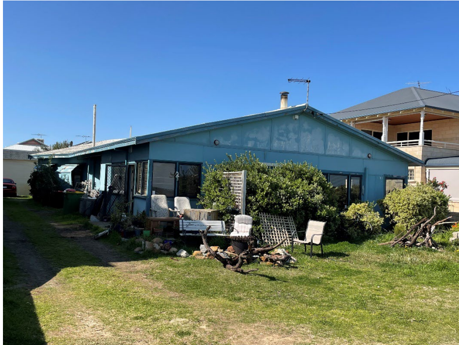
Figure 5: Facade and north elevation
