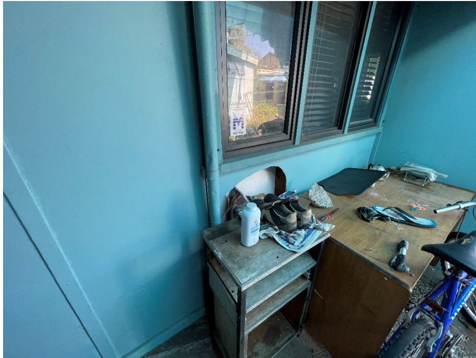
Figure 21: Damaged fibro panelling
