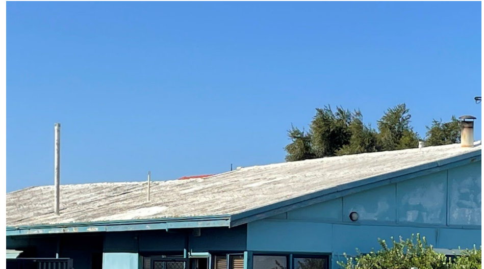
Figure 18: North side of roof taken from street level
