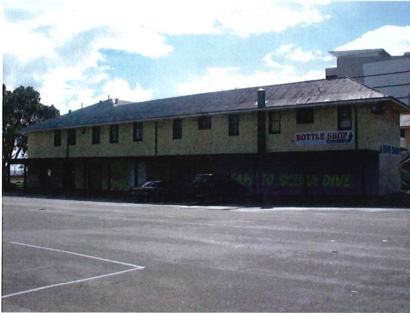
FIGURE 9 SOUTH WEST FACADE Facing carpark (07/07/2008)
