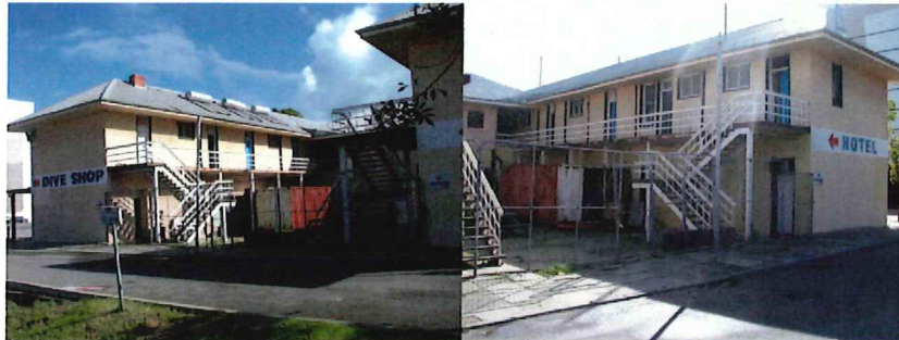
FIGURE 10 A & B SOUTH EAST FACADE Showing U shaped configuration, courtyard, verandahs and stairways. (07/07/2008)
