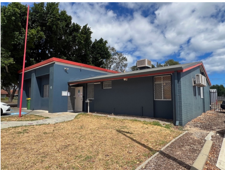
Views of the front (east) facing Hefron Street, and view of the front looking southwest.
