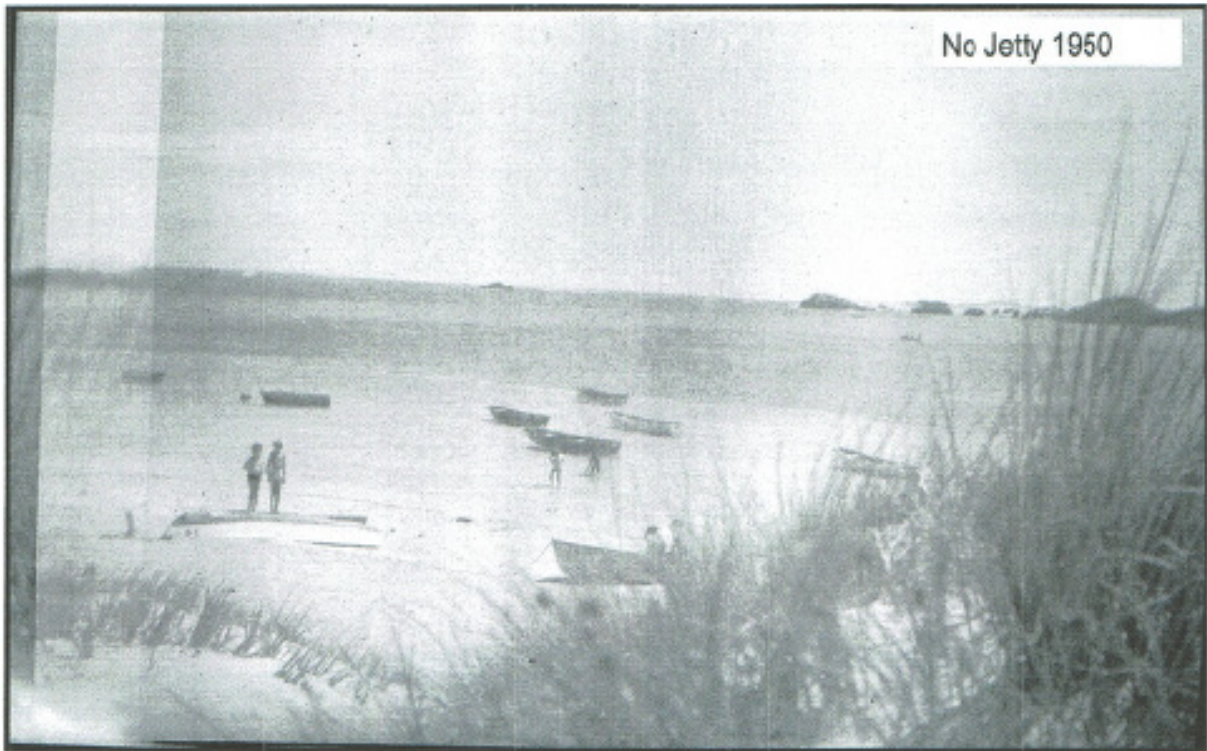
Image of Mersey Point with no jetty in 1950
