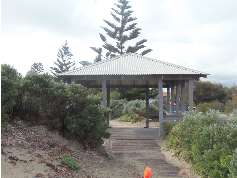
Source: 25 July, 2018. Stephen Carrick Architects
