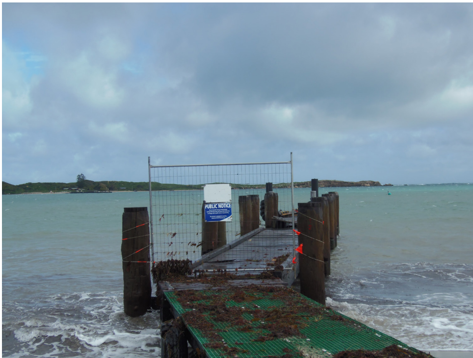
Source: 25 July, 2018. Stephen Carrick Architects
