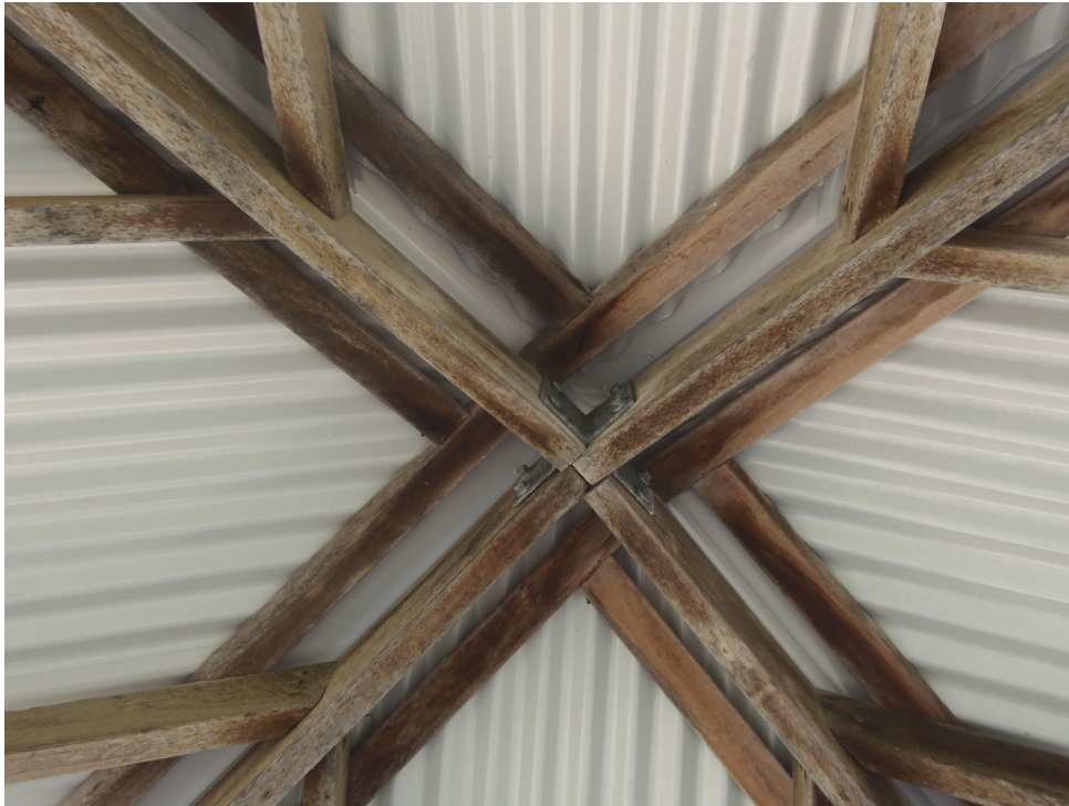
Source: 25 July, 2018. Stephen Carrick Architects
