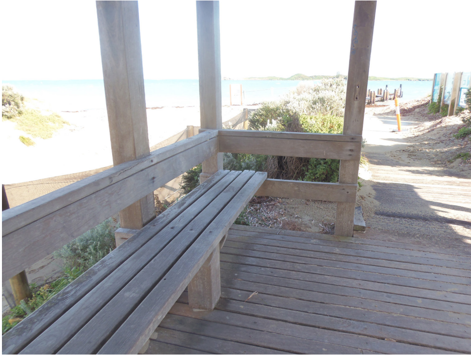
Source: 25 July, 2018. Stephen Carrick Architects
