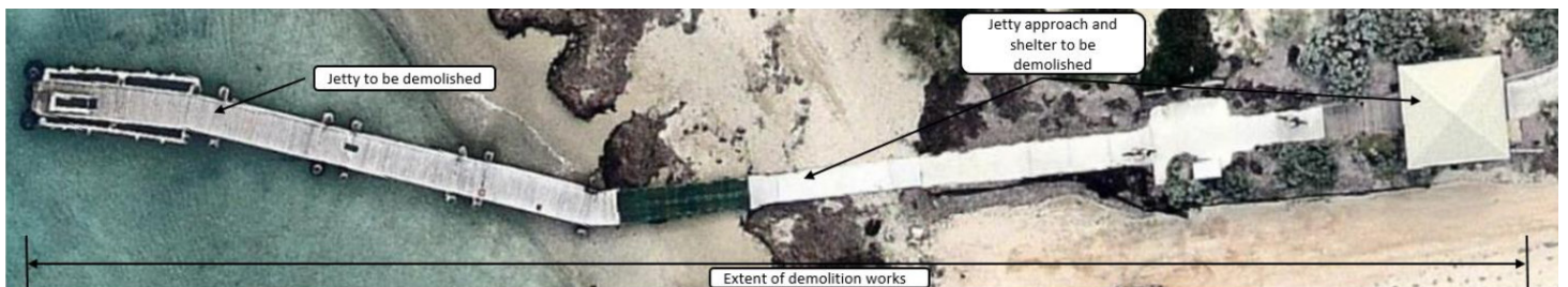
Mersey Point Timber Jetty c2017/18 Image courtesy of Landgate
